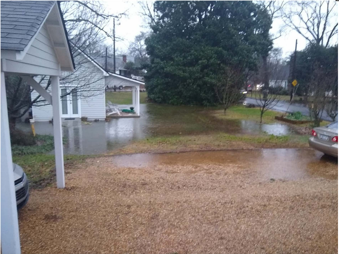
Rain event flooding January 2024
