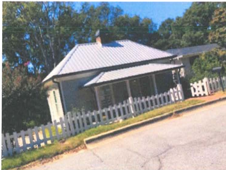
18 Wofford St Wood fence that runs across the FRONT yard:
