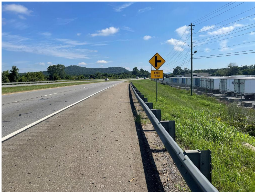
View NE near 1 River Ct.- wide shoulder. Sidewalk begins/ ends in distance
