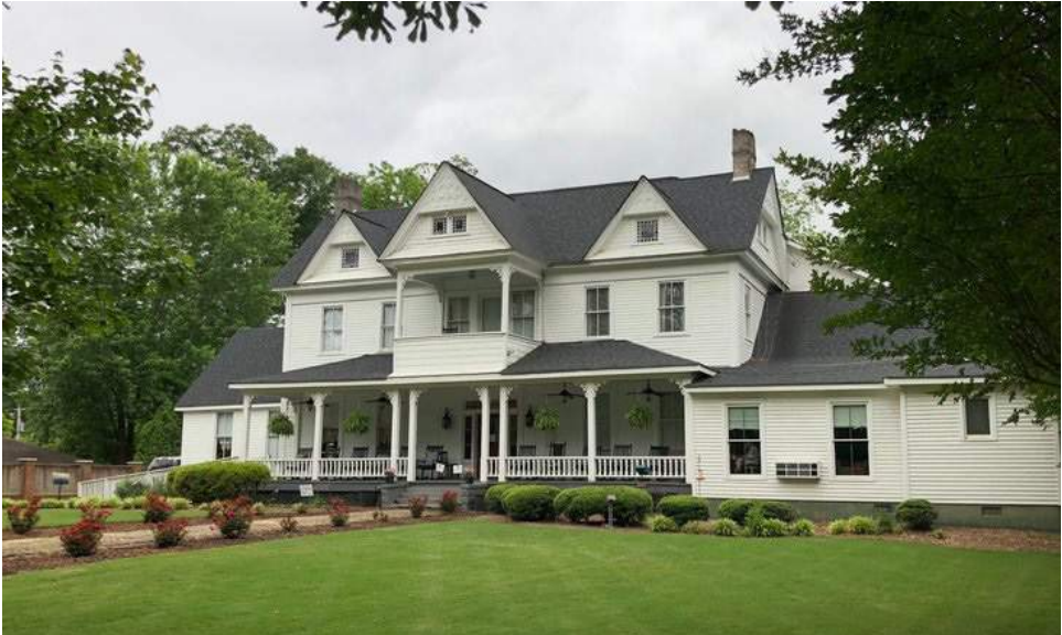
ADJOINING PROPERTY - 5 FITE ST
