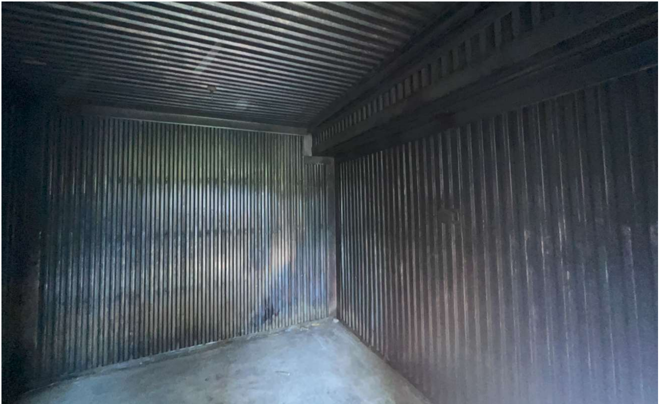
Burn Room #3 Ceiling Panels, Wall Panels & Trims
