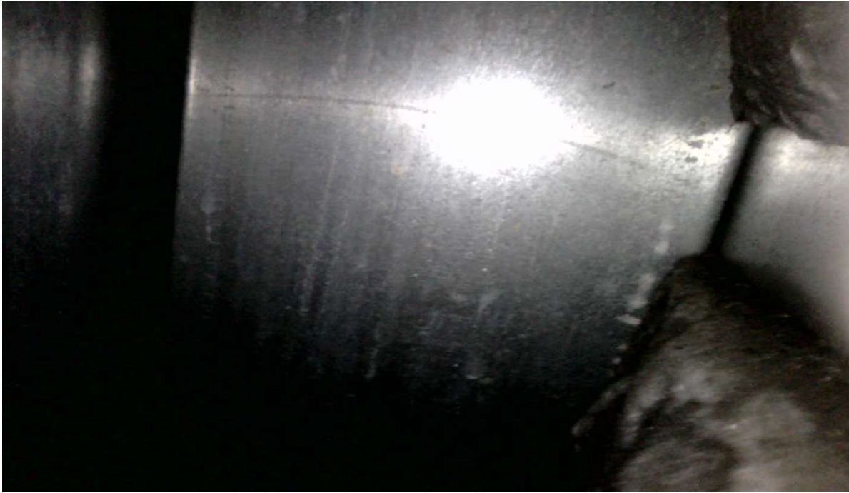
Annex Burn Room – Light Gauge Metal Stud
