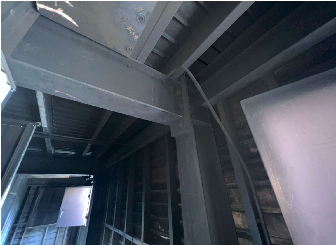
Structural Steel Adjacent to 2 nd Floor Burn Room
