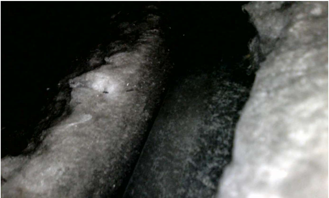
Annex Burn Room Wall Insulation
