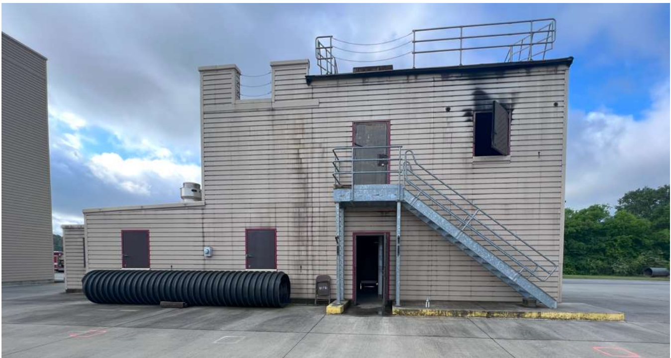
Overall View of the Fire Facilities Inc. Structure
