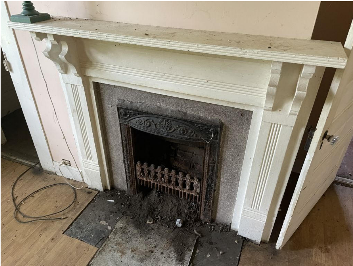
Fire place mantle and cast iron front. Center of House.
