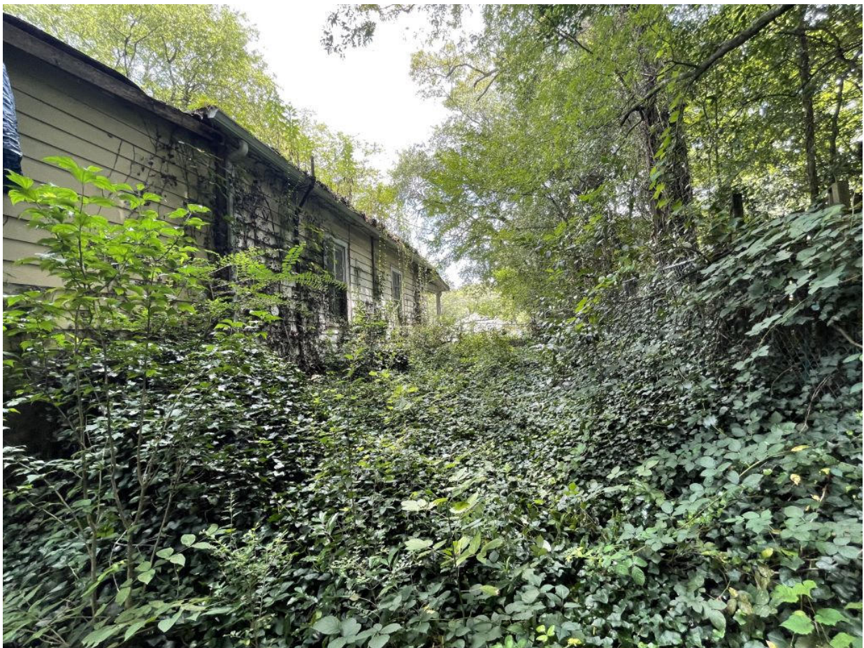
View to south wall from SW corner
