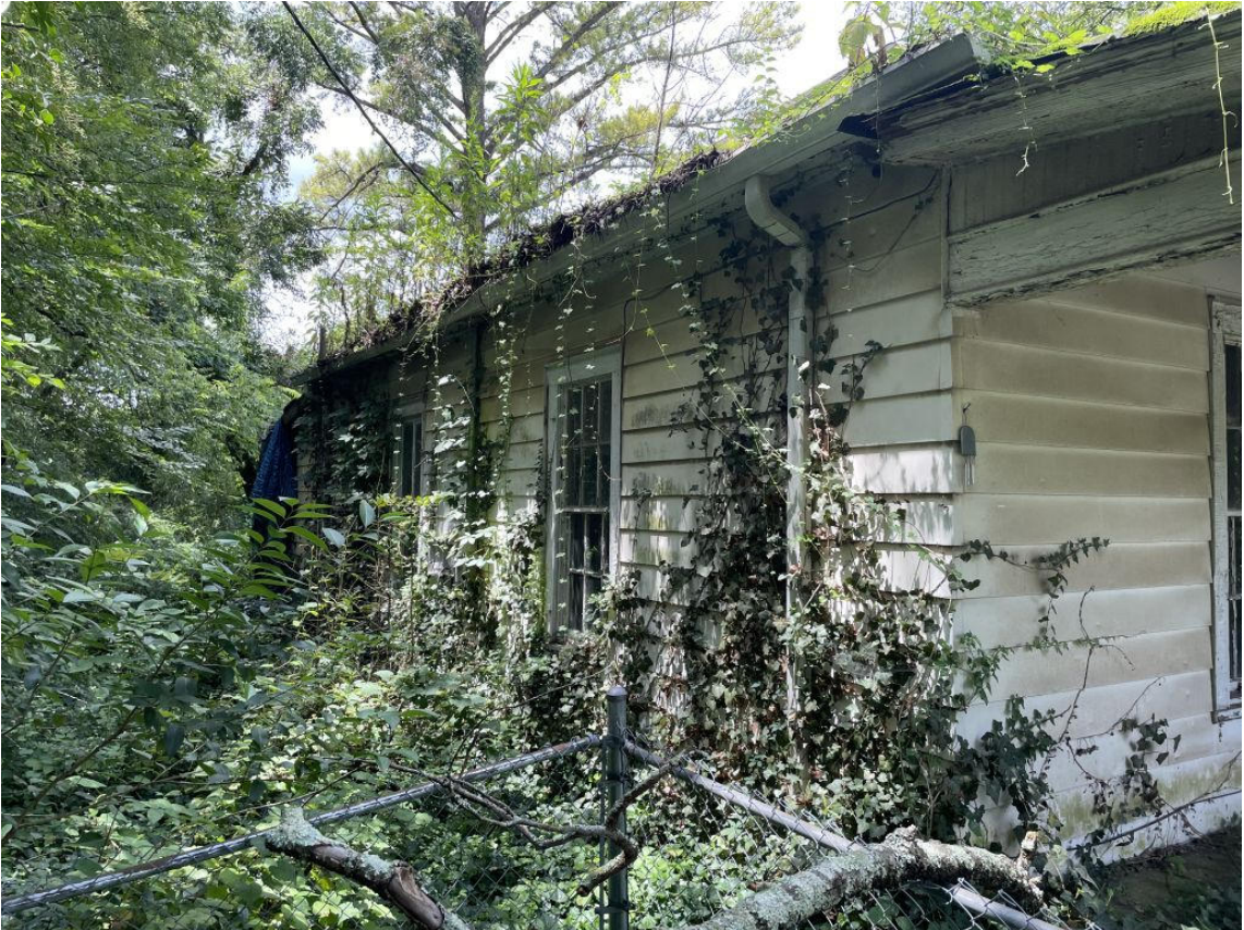
View to south wall from SE corner
