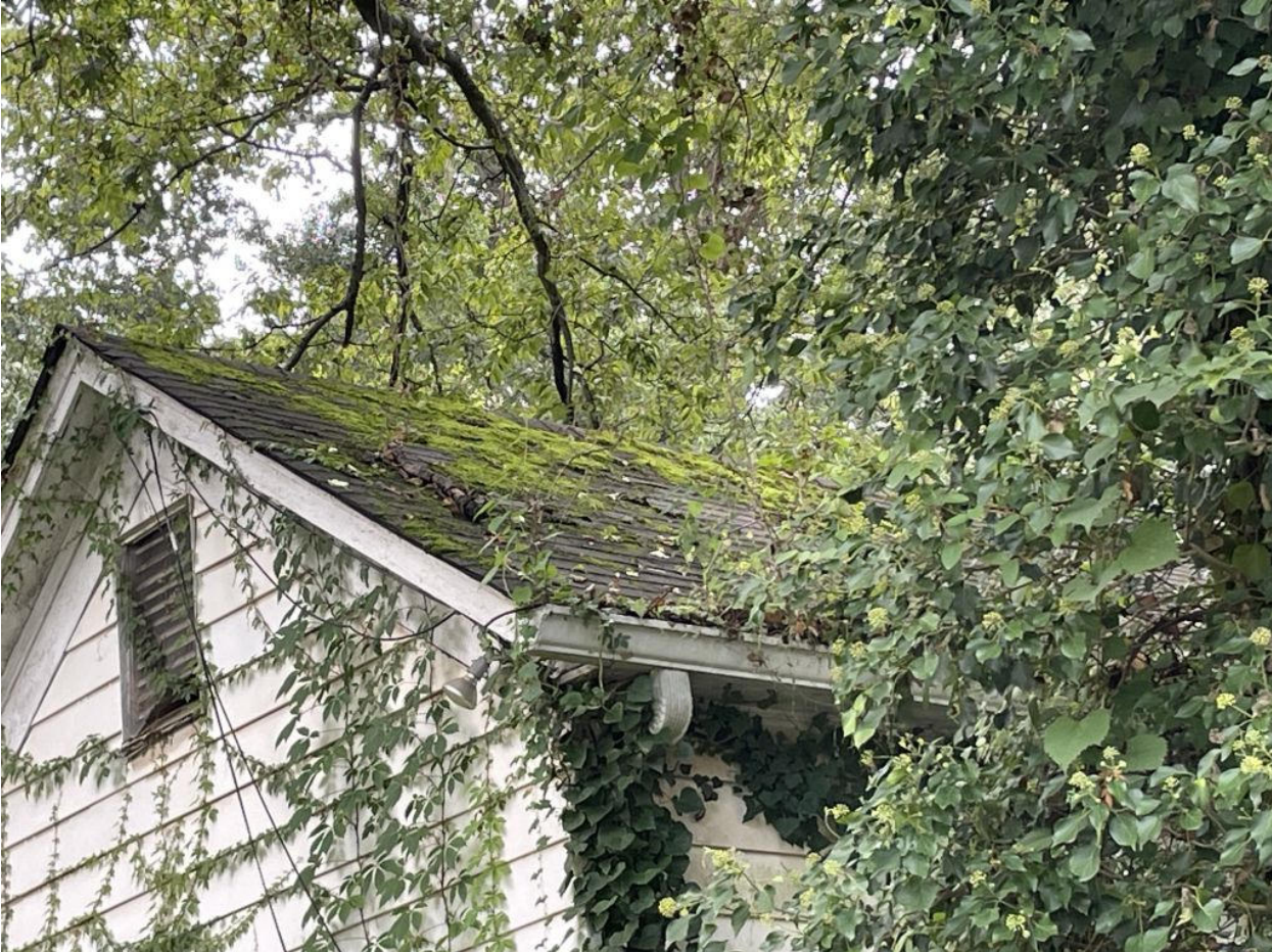
Roof from NE corner.
