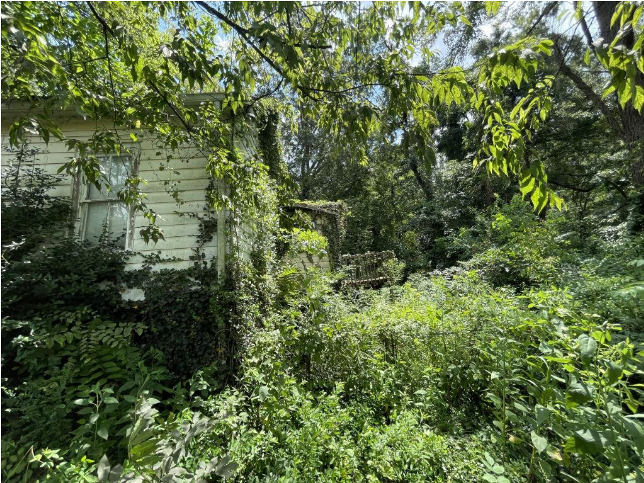
View to rear of home from NW corner
