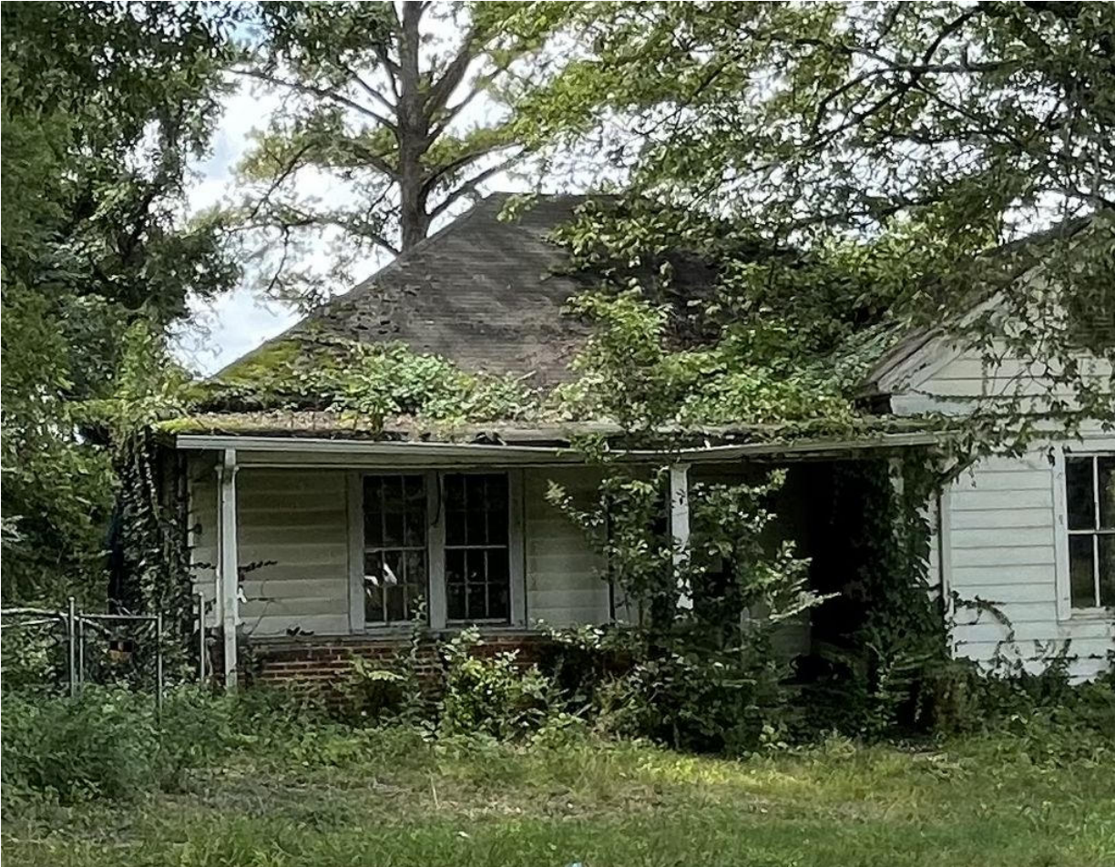
Front of House/ Porch.
