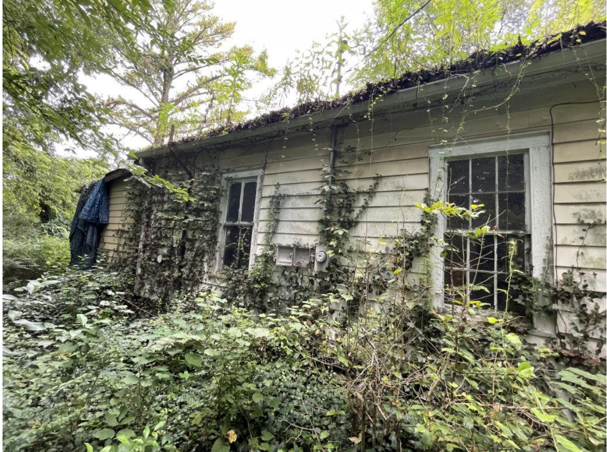
View to south wall from SE corner
