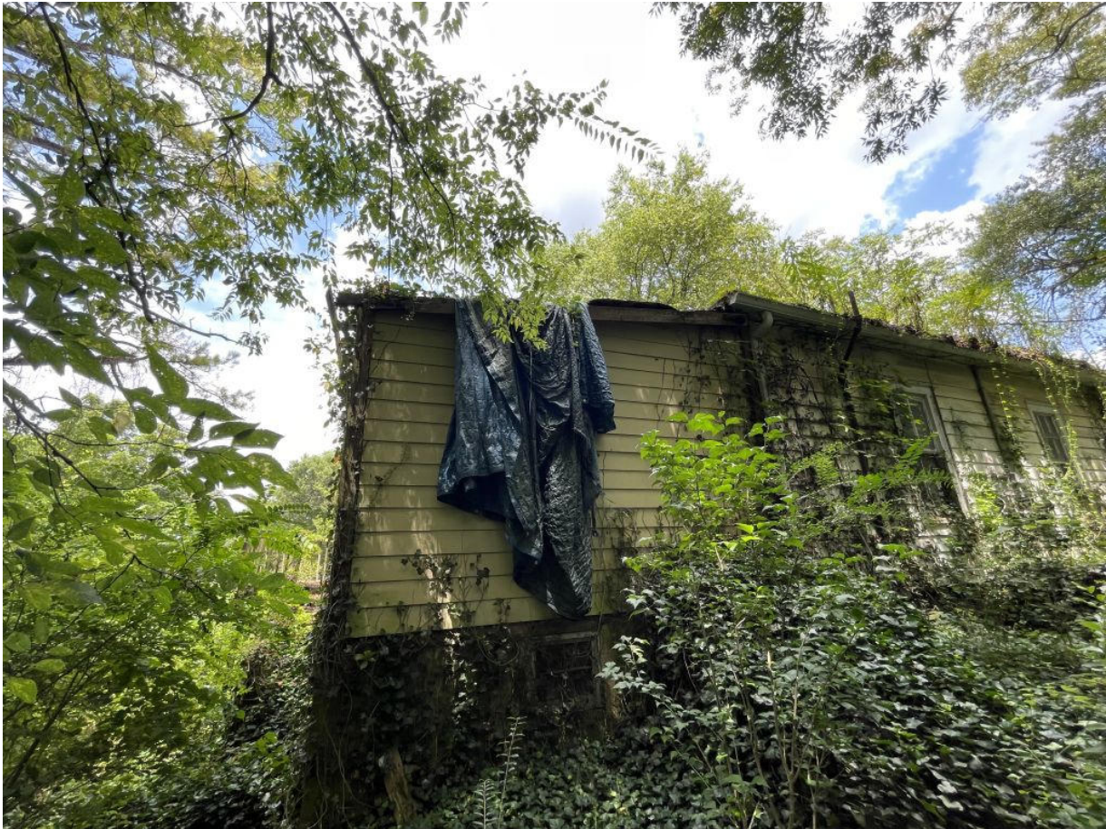
View to south wall from SW corner
