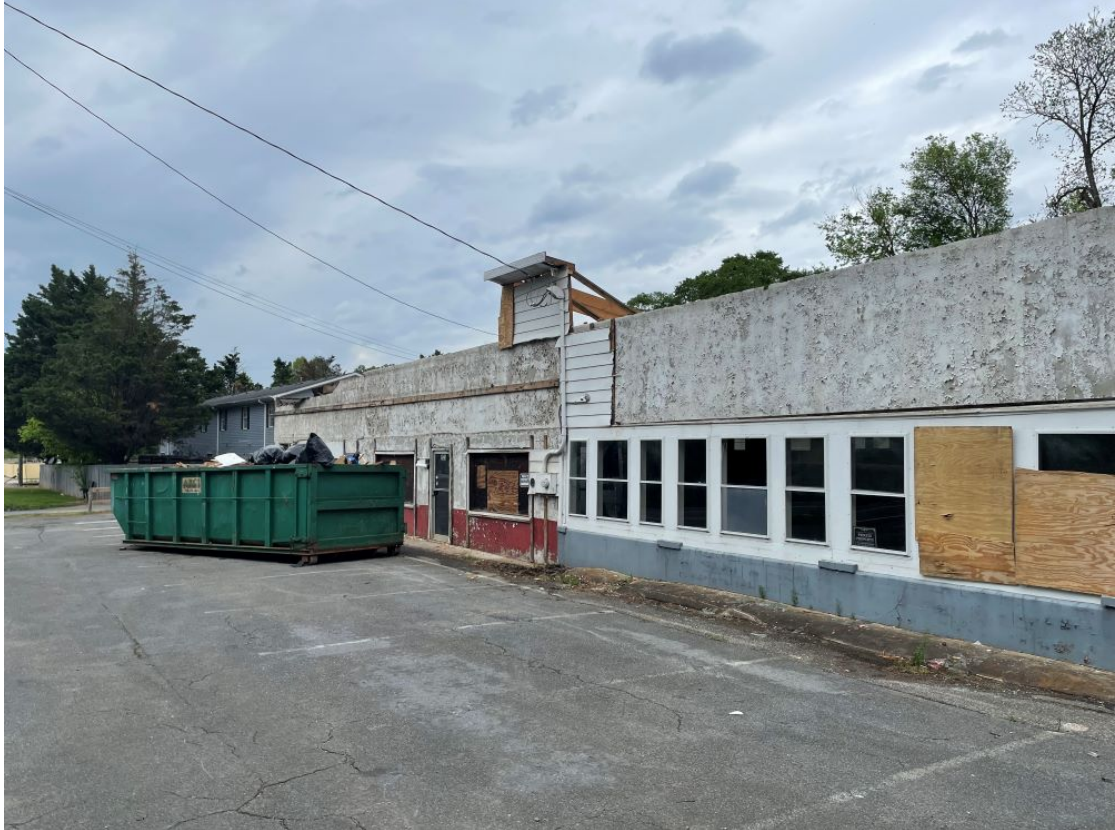
COP22-10. Site Visit on 4-14-23. Interior demolition started.
