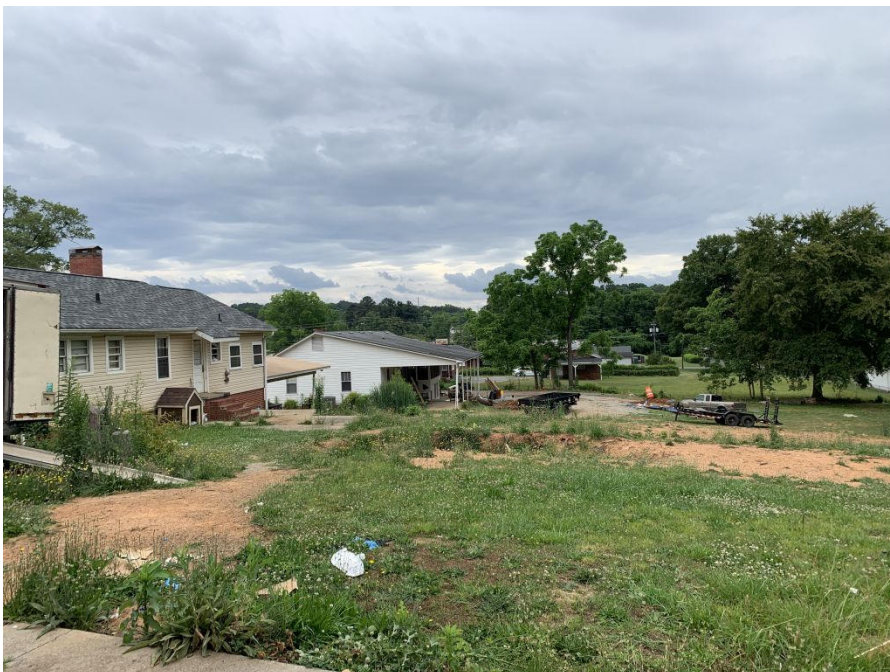
VIEW SOUTH FROM 1010 ACROSS REAR OF 1006 AND 1008 PROPERTIES.
