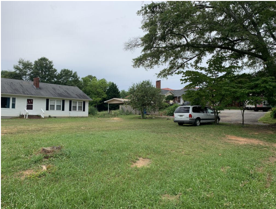
VIEW NORTHWEST TO 1006 AND 1008 STRUCTURES.
