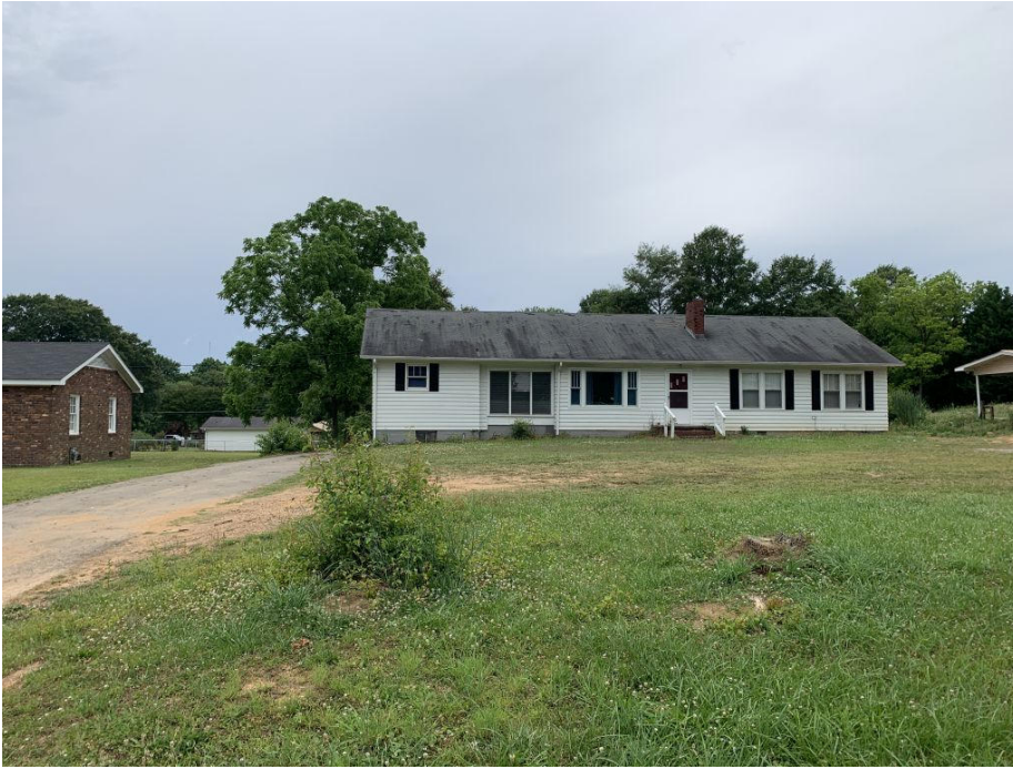
VIEW WEST TO 1006 STRUCTURE.
