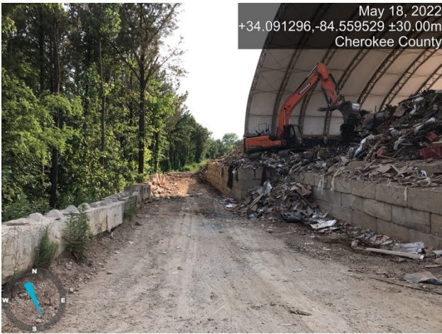
Photo Number: 2 of 4 Date: 5/18/2022 Time: 9:00 AM Weather: sunny Location: Dixie Speedway Transfer Station County: Cherokee Photographer: Jason Rogers Observations: Transfer station operating without confining waste to interior. Station has no floor, only soil beneath the roof
