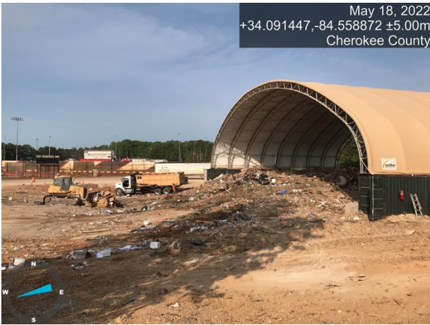
Photo Number: 1 of 4 Date: 5/18/2022 Time: 9:00 AM Weather: sunny Location: Dixie Speedway Transfer Station County: Cherokee Photographer: Jason Rogers Observations: Transfer station operating without confining waste to interior. Station has no floor, only soil beneath the roof.
