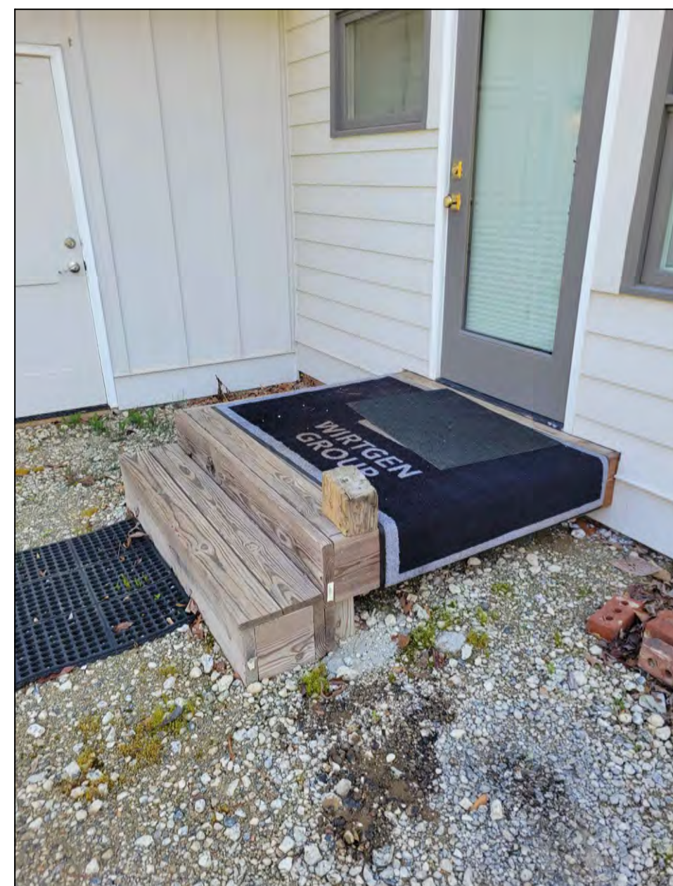
7 OAKLAND STREET BACK DOOR
