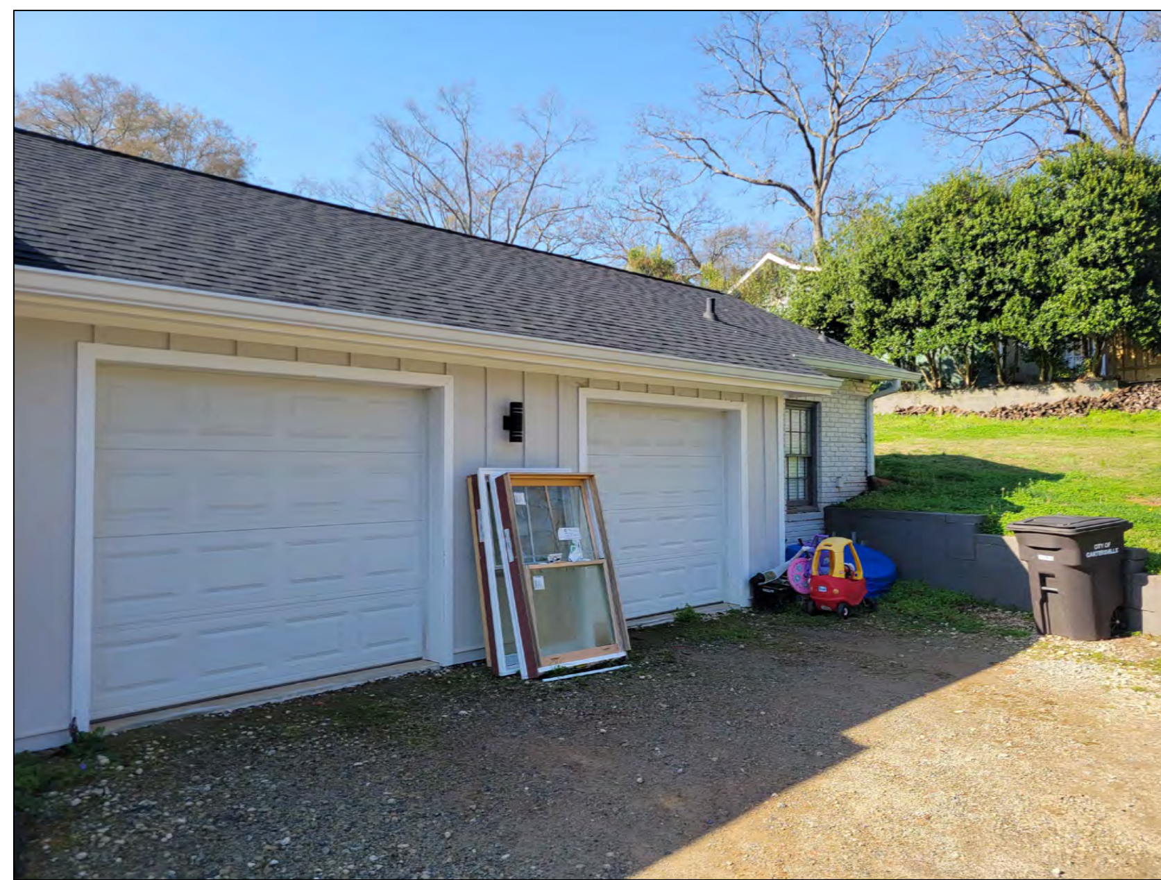
7 OAKLAND STREET EXISTING GARAGE VIEW
