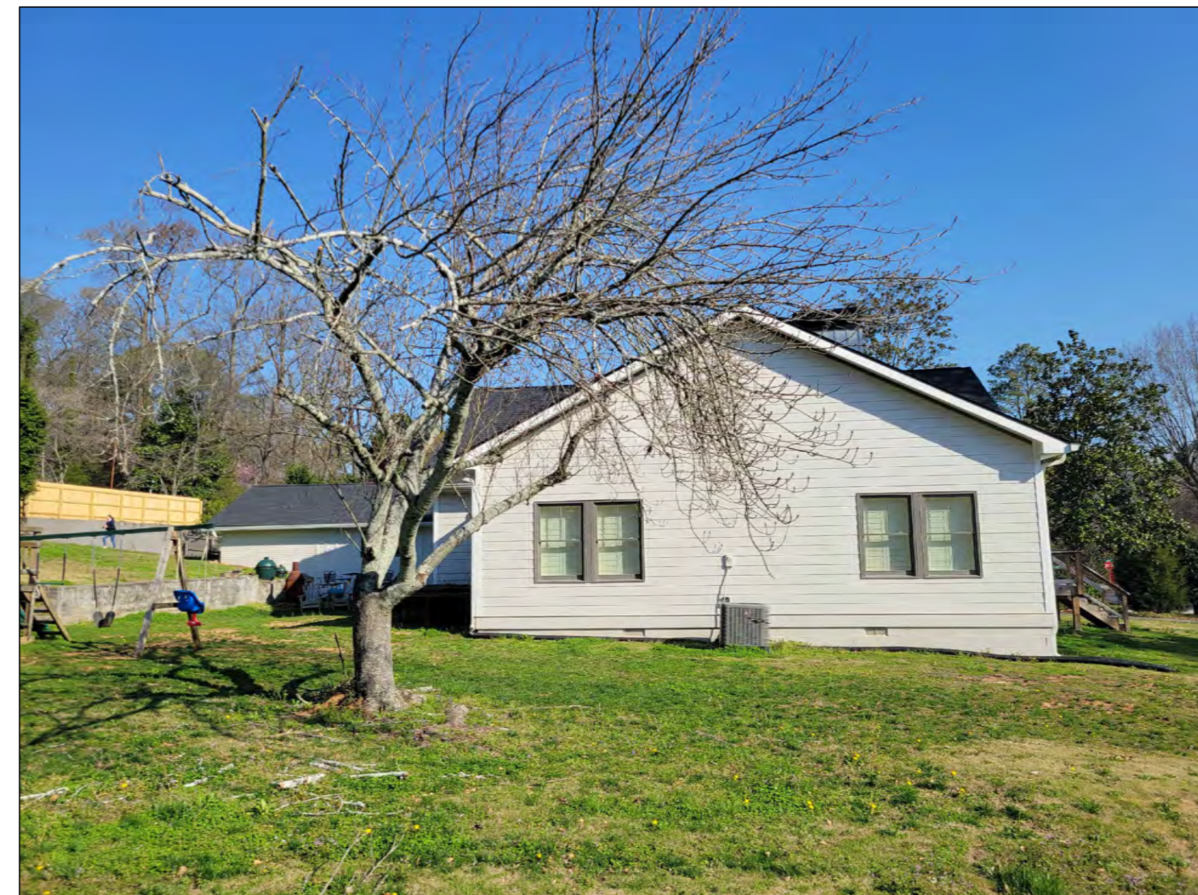
7 OAKLAND STREET EXISTING SIDE VIEW - POPLAR STREET
