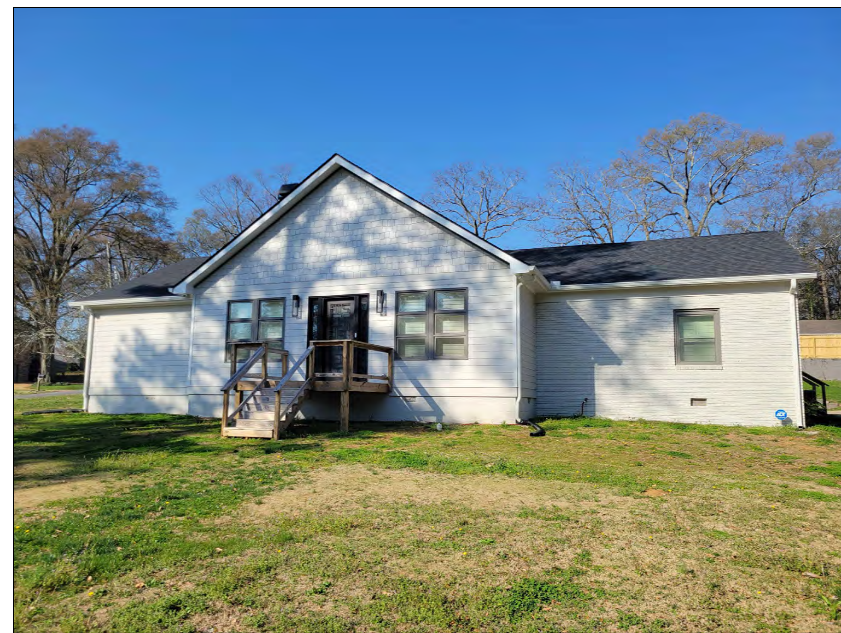
7 OAKLAND STREET EXISTING FRONT VIEW
