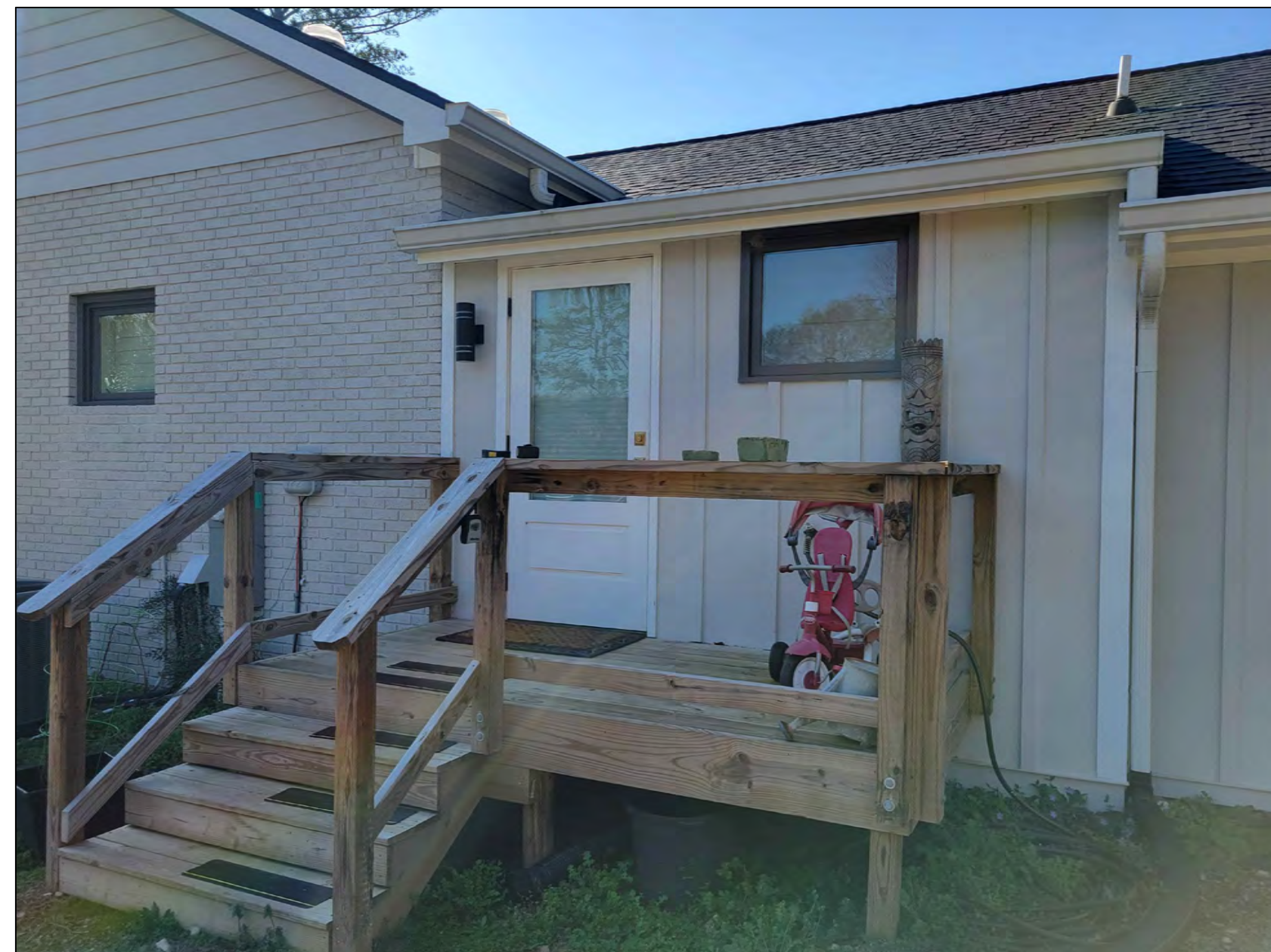
7 OAKLAND STREET SIDE ENTRY VIEW
