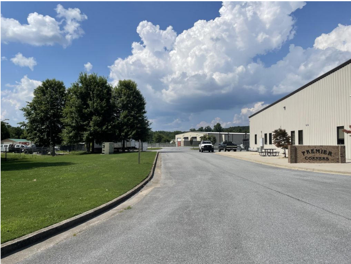
View from Curtis Ct along left side of Building 30. Building 44 is in the distance.
