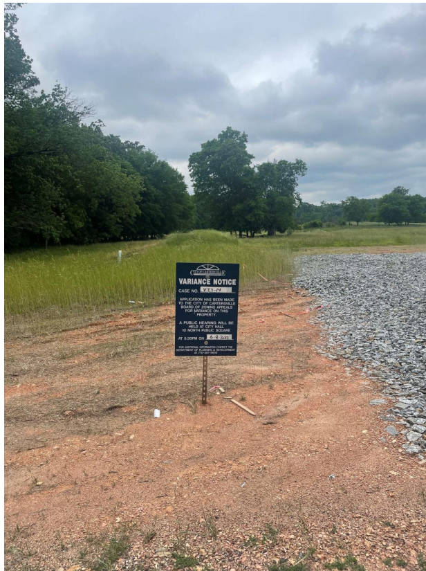
Cass- White Rd Construction Entrance
