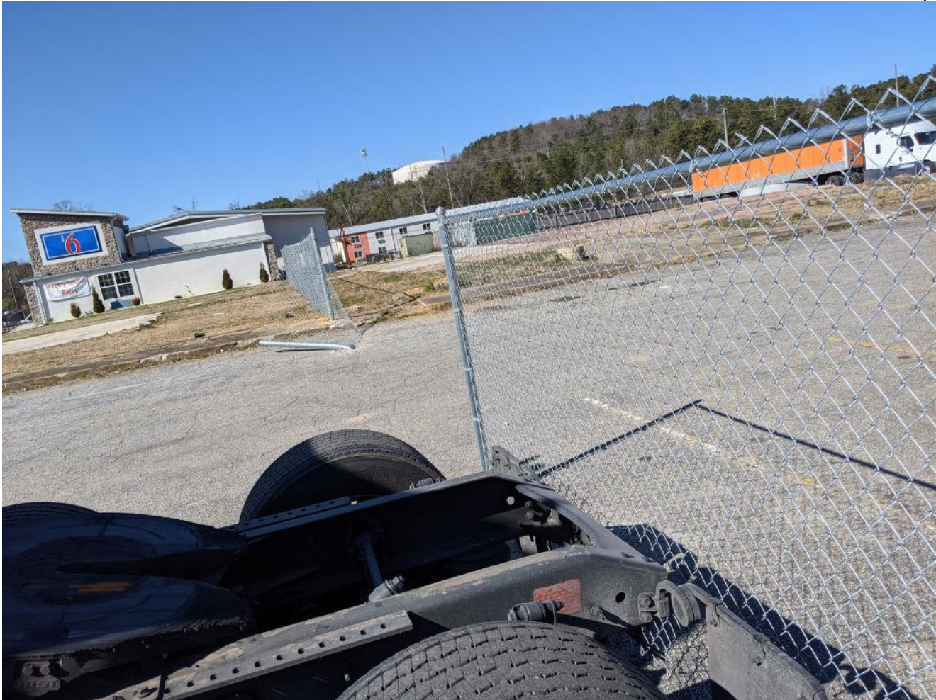
Damaged Fence. Image taken 2-25-21
