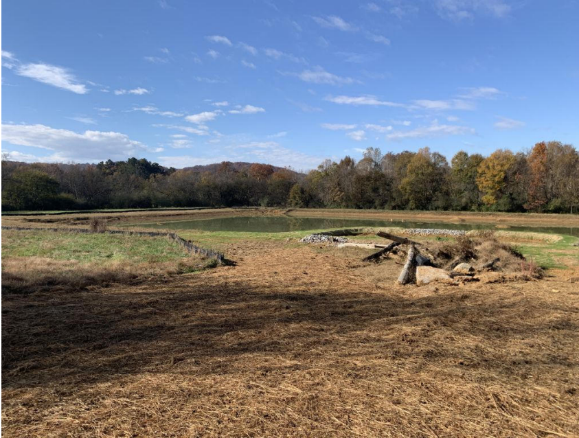
Detention Pond Looking West
