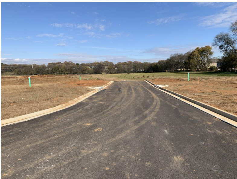
Westover Rd. at Sherwood Rd. looking North towards Phase 2.
