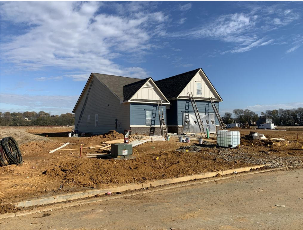
Model Home under construction on Jackson Rd at Silo Dr.
