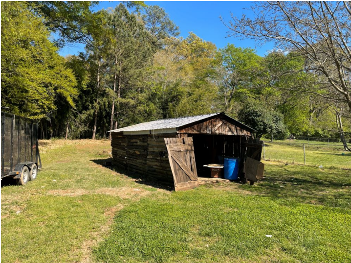
Storage shed to be demolished
