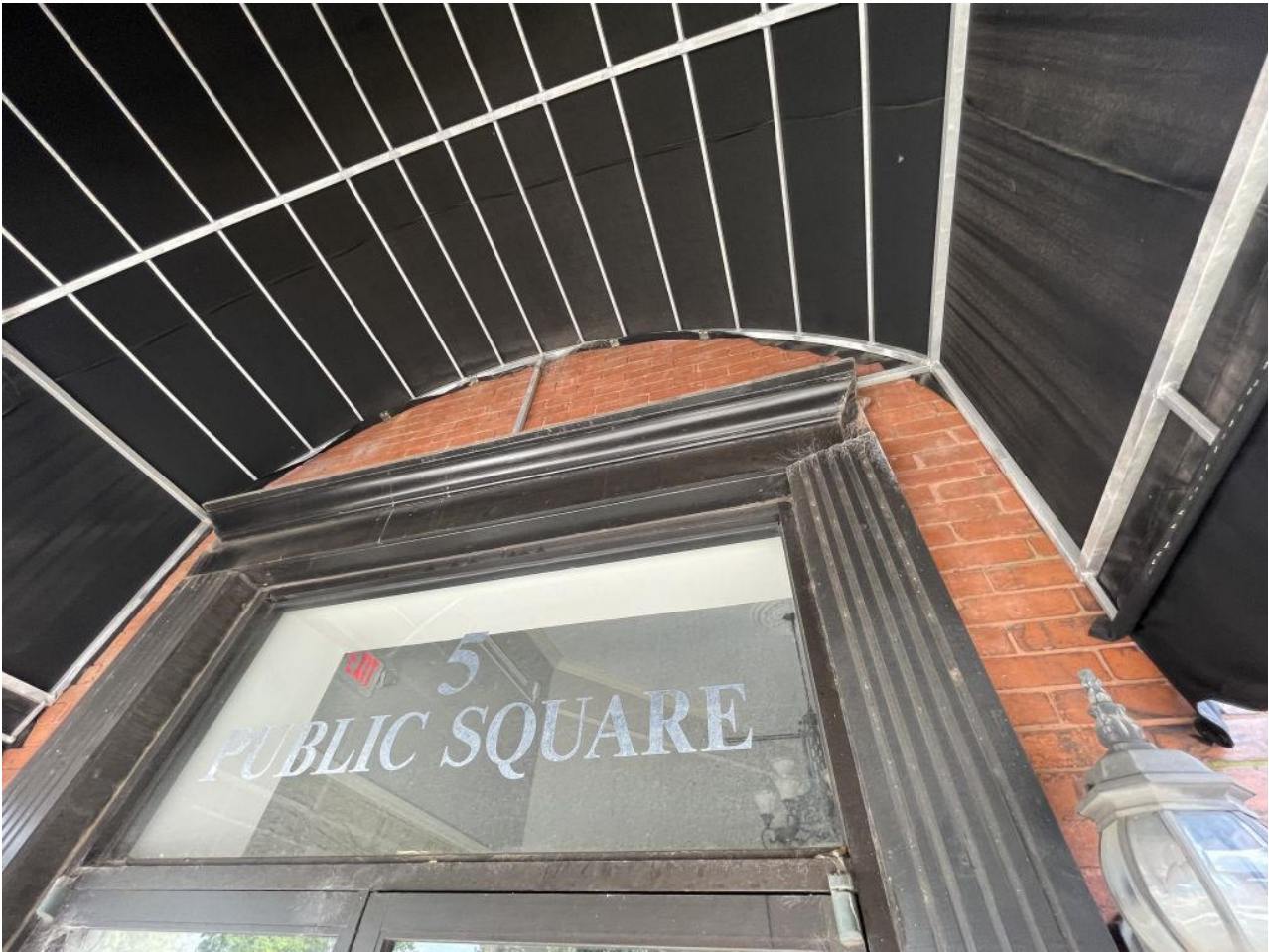
VIEW FROM INTERIOR OF DOORS TO BE REMOVED.
