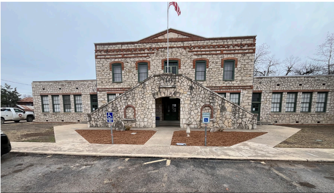
Removal & final grade of the front 2 flower beds.
