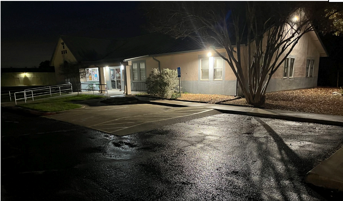
Addition of 2 new LED lights on the Library Building.
