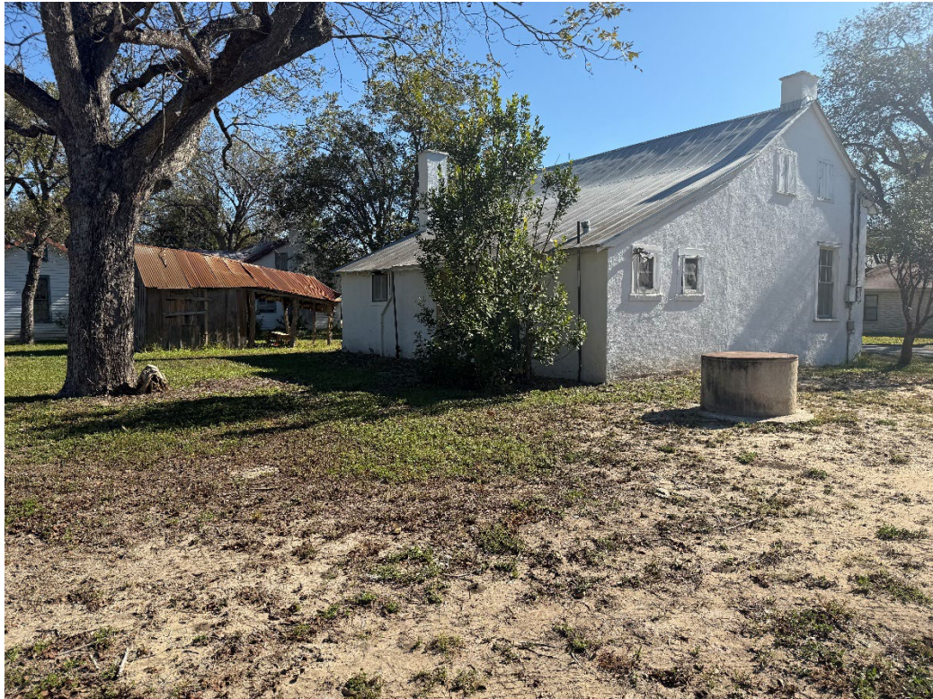
Rear/North Side of House: These 3 images show the location of the pecan tree and well. Along the north side, we will be adding on a full kitchen and dining space, as well as an outdoor patio along the back of the house. The well will be located inside the addition and cut down to floor level so you can walk over and see down it.
