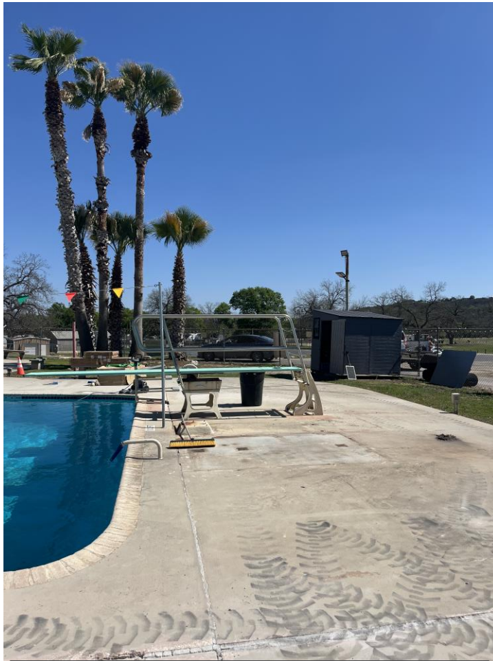
Removal of the three-meter diving board & platform. Next Steps: Move the one-meter board to the center of the diving well.
