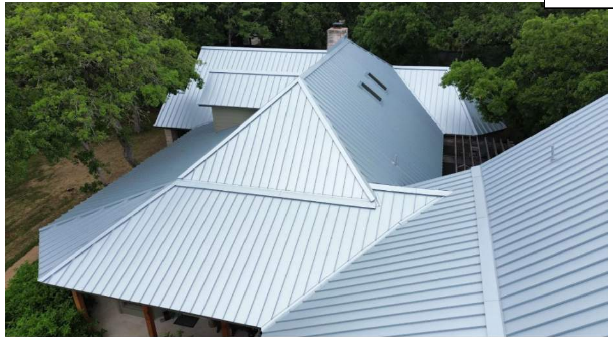
24 gauge glavalume standing seam metal roof
