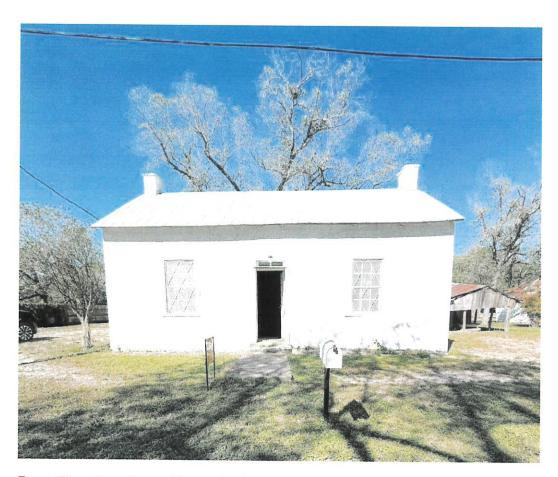
Front Elevation: This will remain the same, other than replastering and removing of the aluminum window screens that take away from the original windows. A light will also be added next to the front door and a new concrete landing/uncovered patio across the front of the house (this is shown in the plans and will not have a roof over it)
