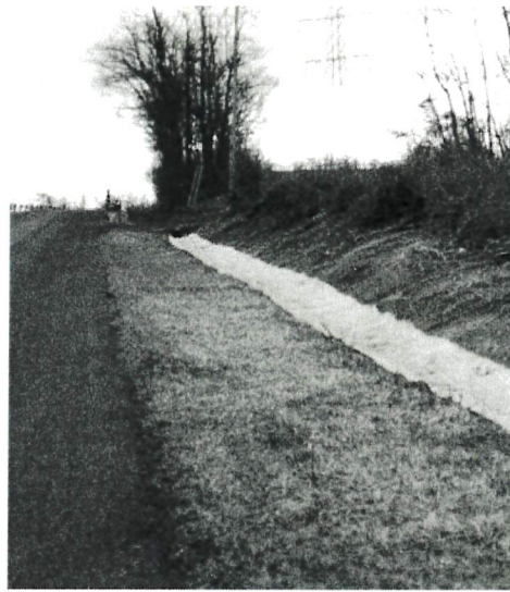
Erosion control measures such as fiber mats shown may be necessary to prevent ditch erosion.
