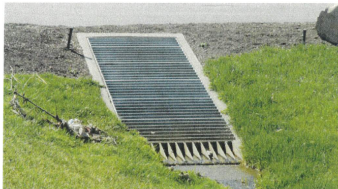
Grated inlet flush with ground over a culvert end.
