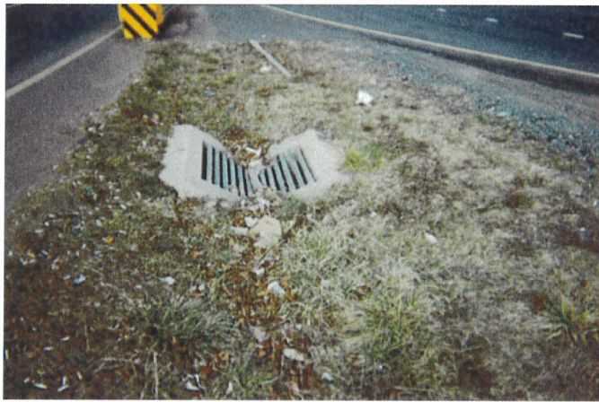
V-shaped grate in median.
