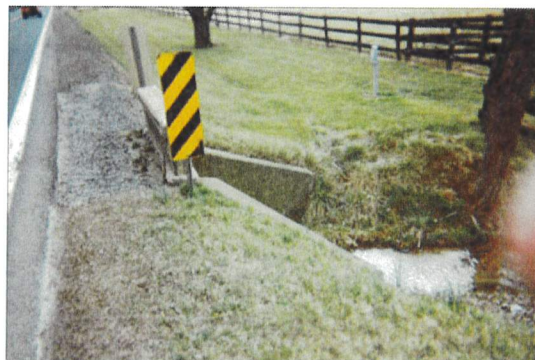
Rigid headwall delineated with Type 3 Object Marker.
