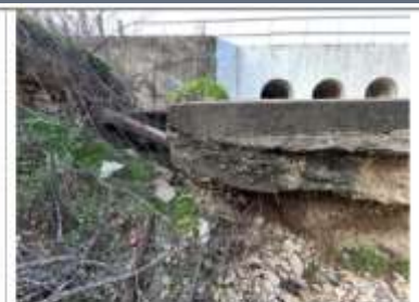
5b – Geneva Street culvert showing scour erosion, undermining of the concrete apron to a cantilevered condition, exposure of water line. (Facing upstream)
