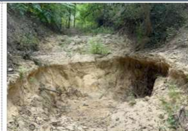
3 – Channel degradation. Deep incision due to steep channel bottom and constriction of flow resulting in increased velocities. (Facing upstream)
