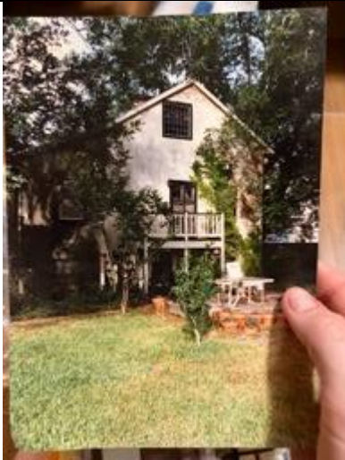
Repair of stucco to match existing historic texture and finish
