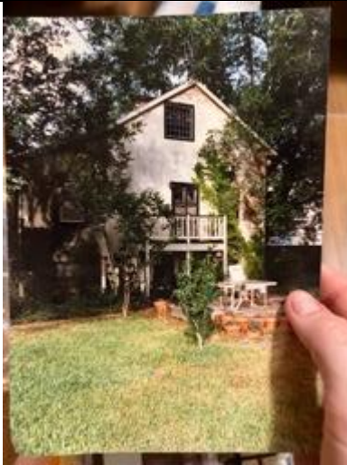
Reconstruction of the historic porch and stair configuration on side of the home based on archival photographs
