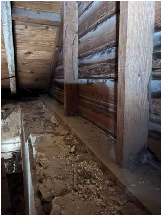
Photos of the inside of the southeast gable end. The wood plate at the top of the stone wall matches the other wall plates and the studs are the same species and vintage of the original roof rafters.
