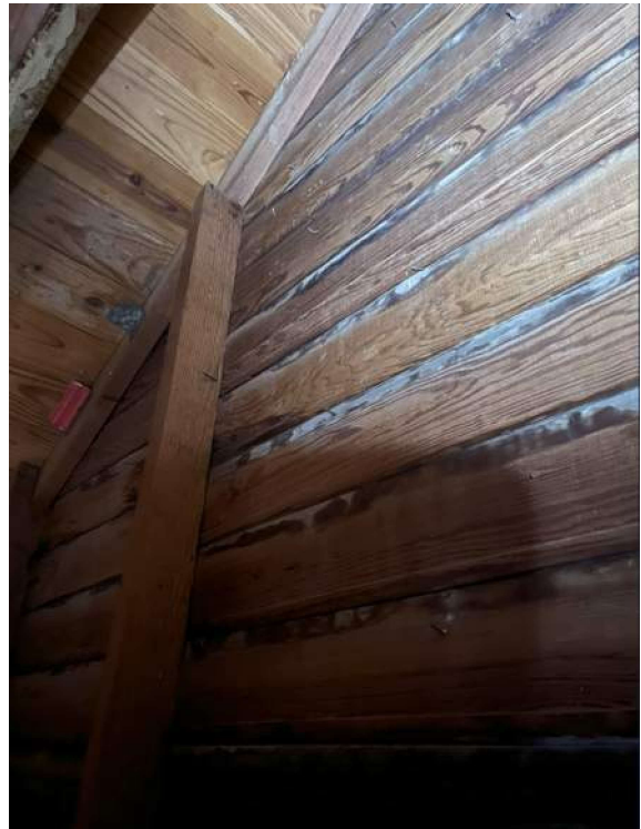
Photos of the inside of the southeast gable end. The wood plate at the top of the stone wall matches the other wall plates and the studs are the same species and vintage of the original roof rafters.
