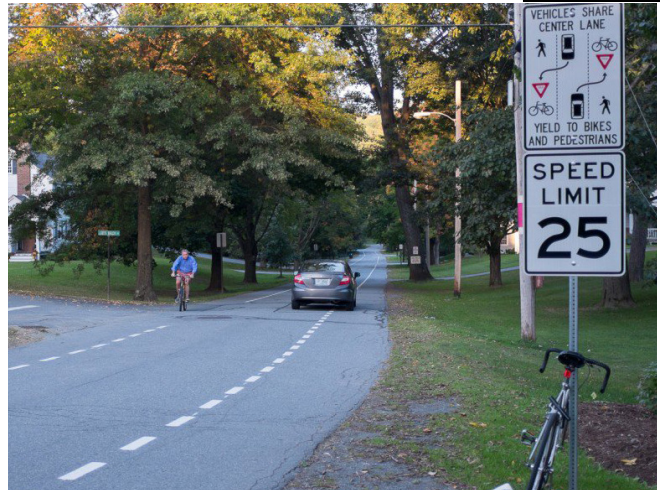
Advisory Bike Lanes could be implemented along Old Highway 90 and County Road 4711 as a first step in the implementation process to accommodate bikers and walkers on existing infrastructure.
