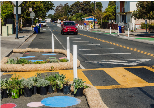
Temporary curb extension demonstration project.
