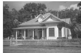
"High-style" residential style, in this case a Queen Anne cottage in an "L-plan" shape, (c. 1909).
