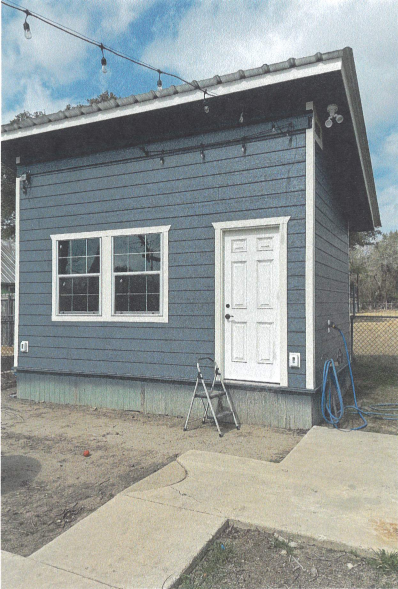
current state of building 3/4/26
