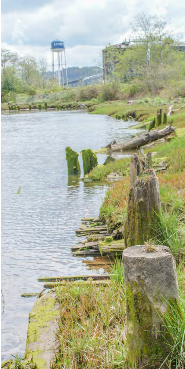
Existing Cosmopolis shoreline along the Chehalis River (Source: Stantec)
