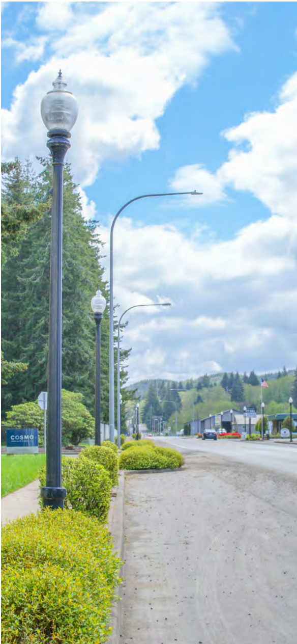
Highway 101 (1st Street) streetscape (Source: Stantec)
