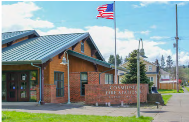
Existing Fire Station building (Source: Stantec)
