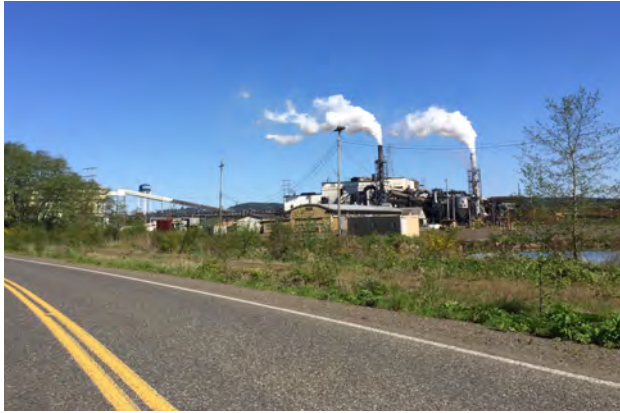
Cosmo Specialty Fibers mill facility (Source: Stantec)
