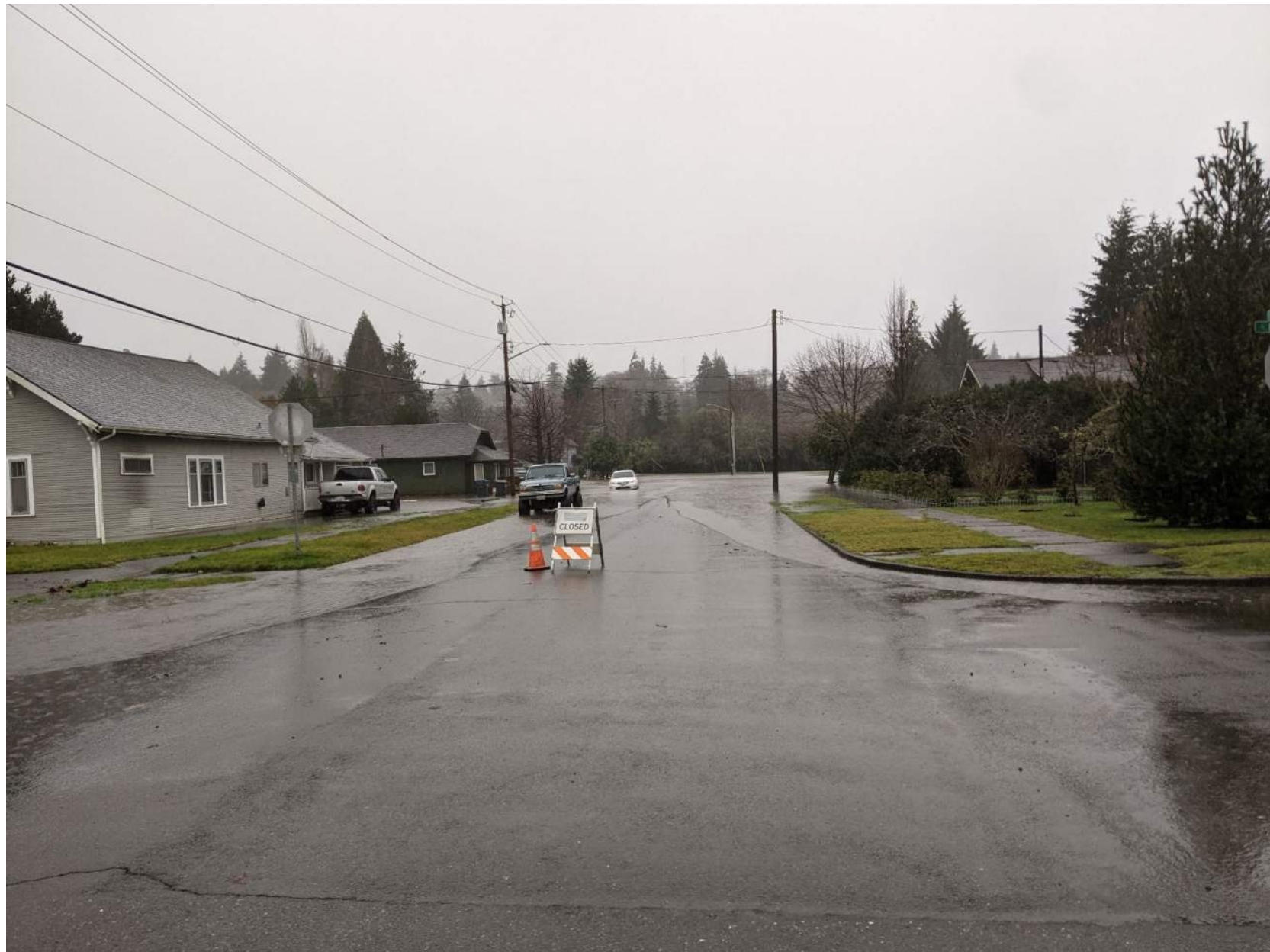
Figure 2. Flooding at 4th and I St Intersection
