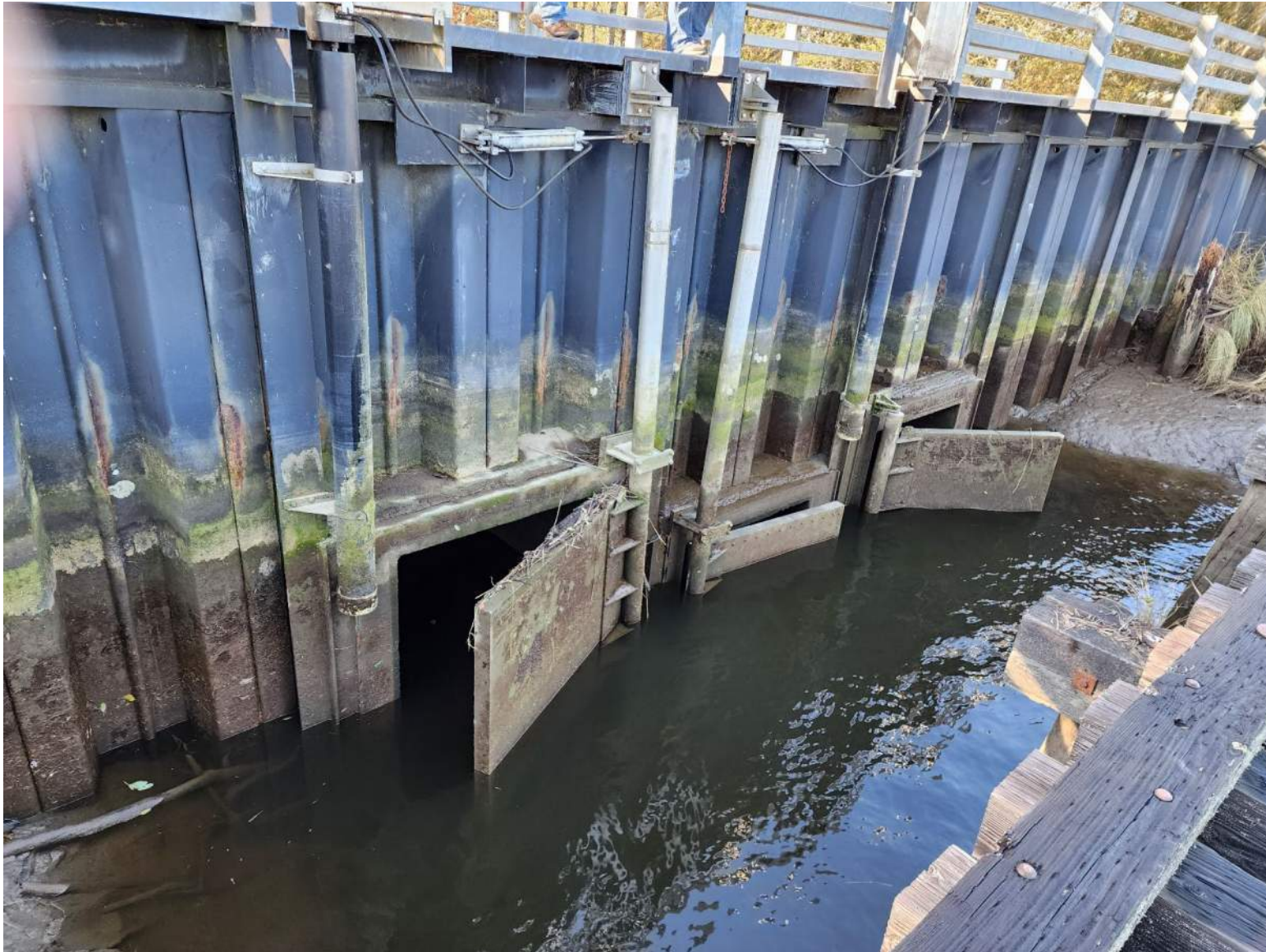
Figure 2. Existing Tide Gates (Downstream side)
