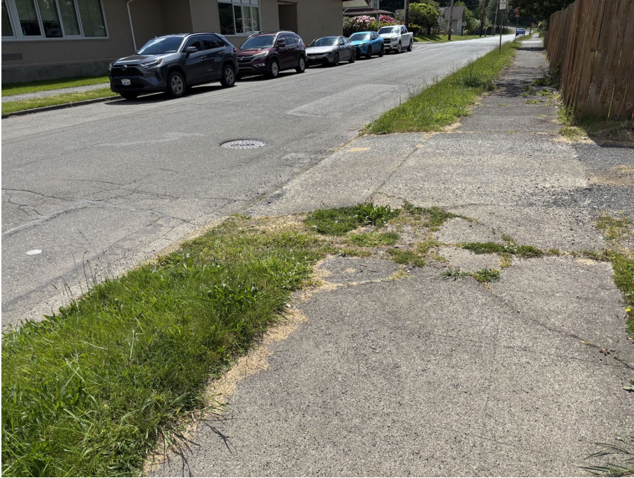
1. C Street sidewalk between 2 nd & 3 rd St.
