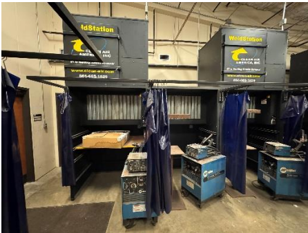
B: Welding Booths
