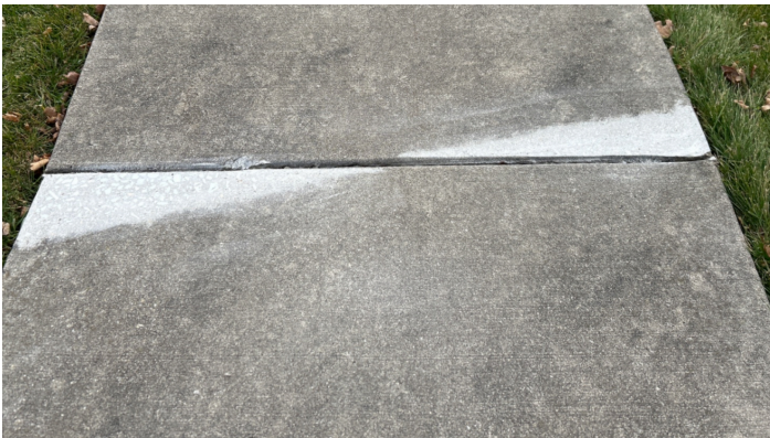
Sample Repair Photo: Defect 392 repaired on 12/21/23 at 16038 Arborvitae Circle.
