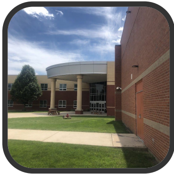
“Filled” New Building
