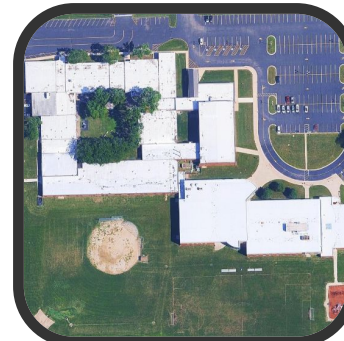
Multi-Million Roof Repairs
