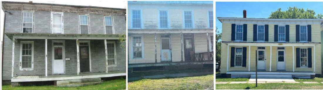
On left, original look of the duplex structure.
