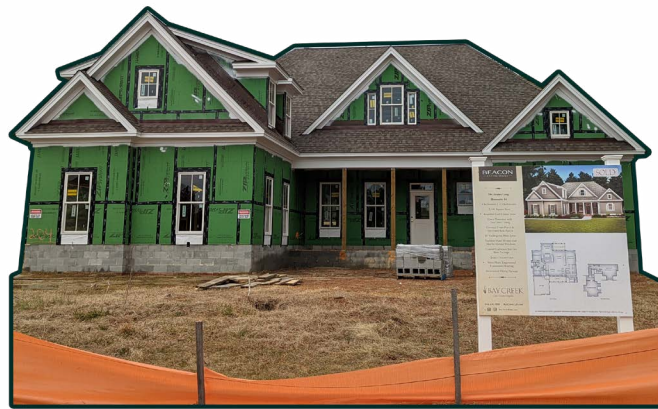
Home under construction in Bay Creek.
