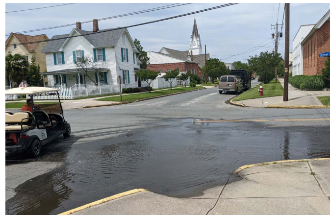
A golf cart drives past pooled stormwater.
