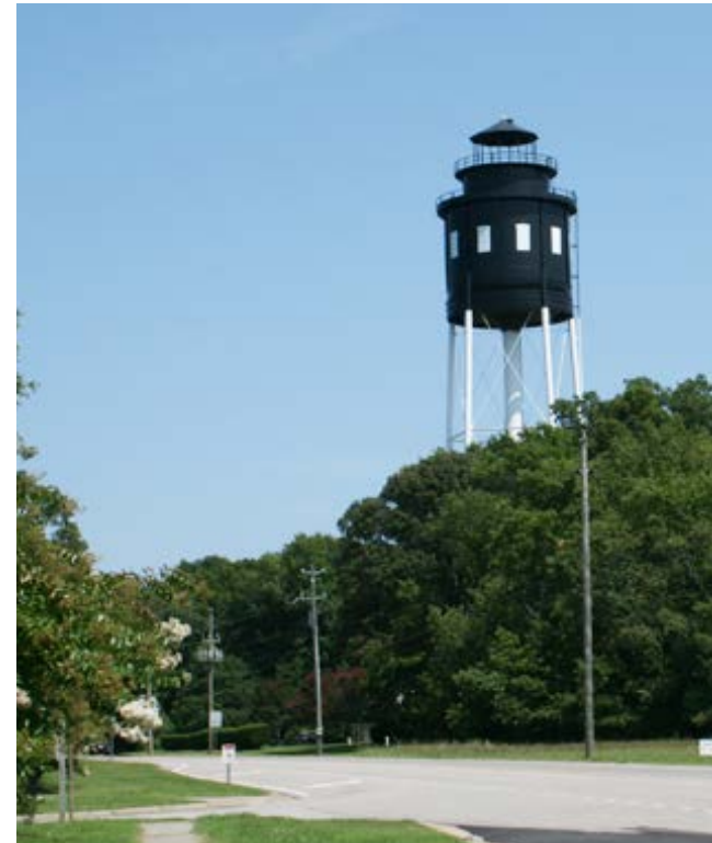
Cape Charles water tower.
