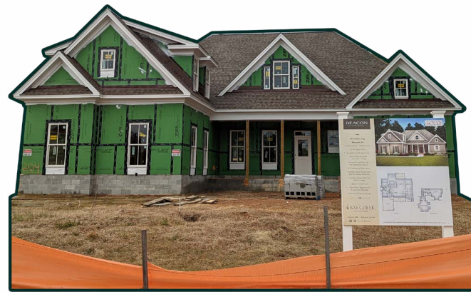
Home under construction in Bay Creek.
