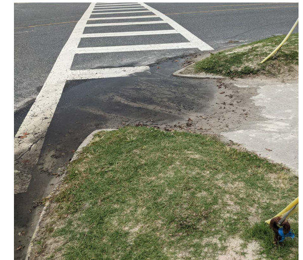
Storm water at a Mason Ave. crosswalk.
