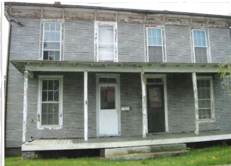
On left, original look of the duplex structure.
