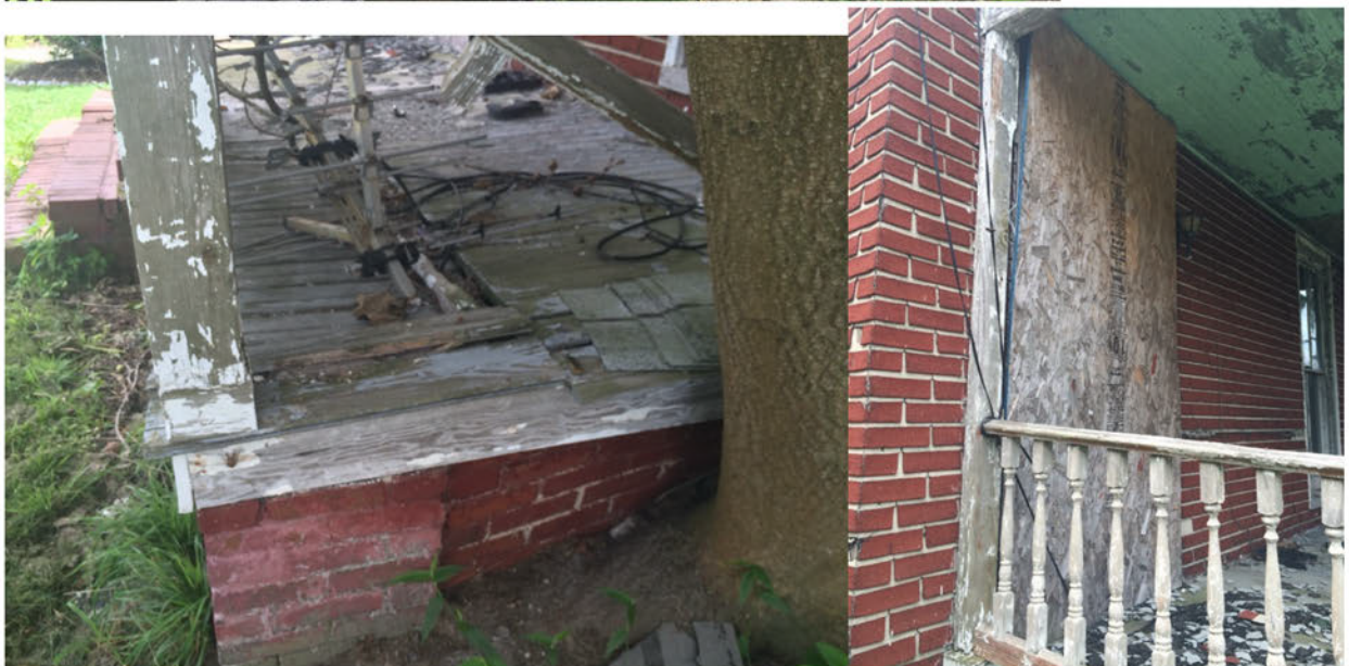
Photos from 2015 before initial renovation.
