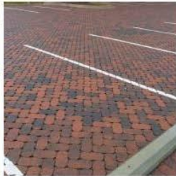
Permeable brick paving
