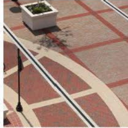
Mix of paving patterns with brick colors
