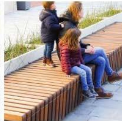
Wood slat benches integrated into seat wall
