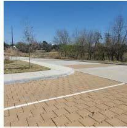
Pavers used for parking bays
