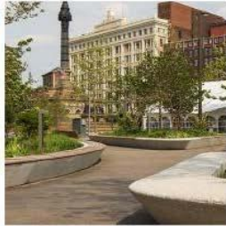
Cast in place concrete seat walls
