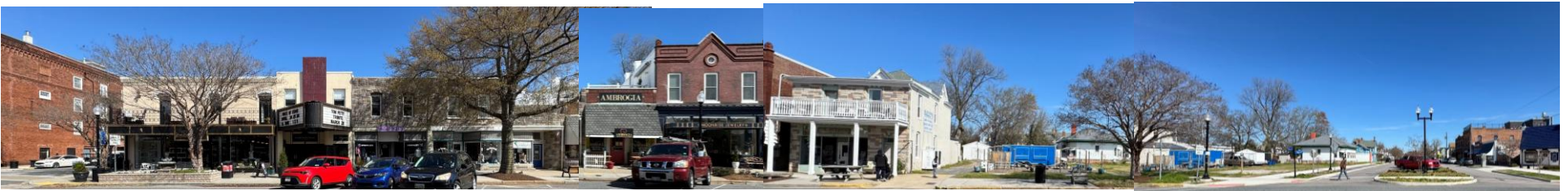
4. Mason Avenue, south elevation, between Strawberry Street and Peach Street
