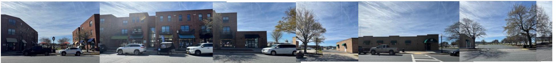
3. Mason Avenue, north elevation, between Strawberry and Pine Streets
