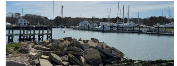
View facing south side
