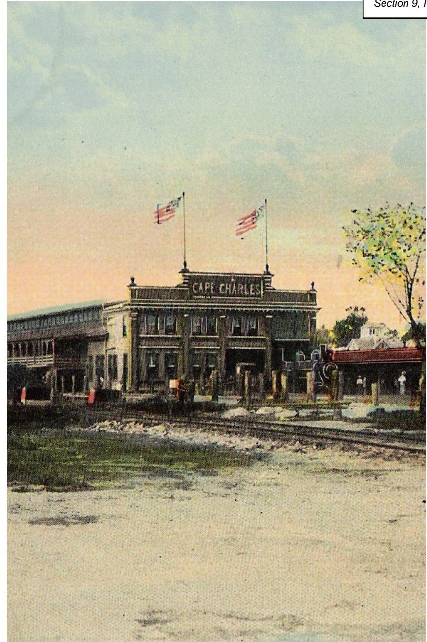
Cape Charles Harbor Terminal Building, 1911.
