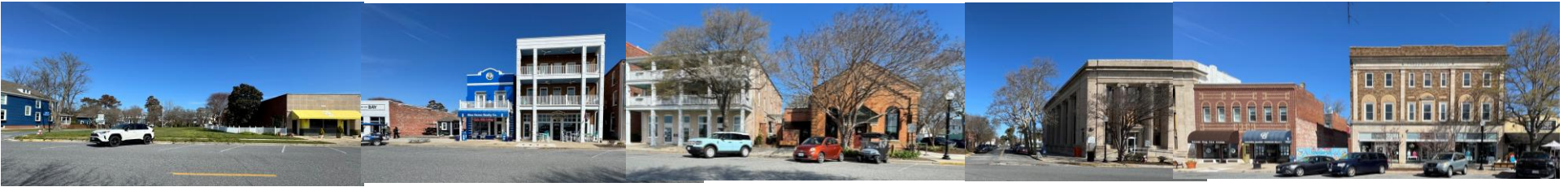
2. Mason Avenue, south elevation, between Harbor Avenue and Pine Street
