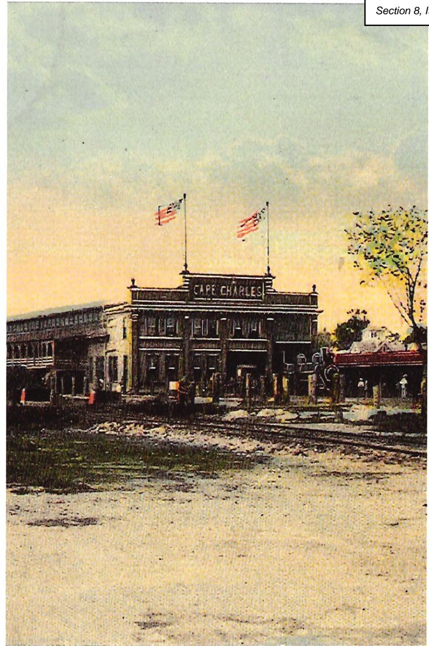
Cape Charles Harbor Terminal Building, 1911.
