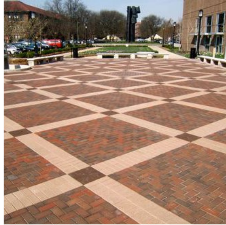
Cross Pattern Brick Paving
