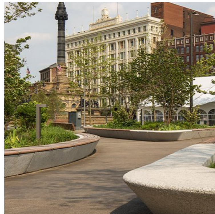
Cast in place concrete seat walls
