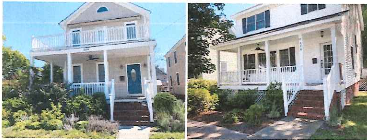
548 Madison. Tooled support columns, but squared railings/balustrade posts. +spindles
