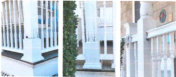
Rotting Porch Columns: Left, Left Center, Right Center
