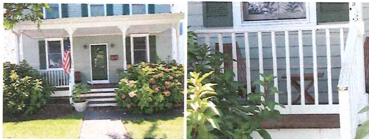
548 Madison. Tooled support columns, but squared railings/balustrade posts. +spindles
