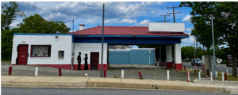
Building at Bladensburg Rd and 38th Ave, proposed visitors center
