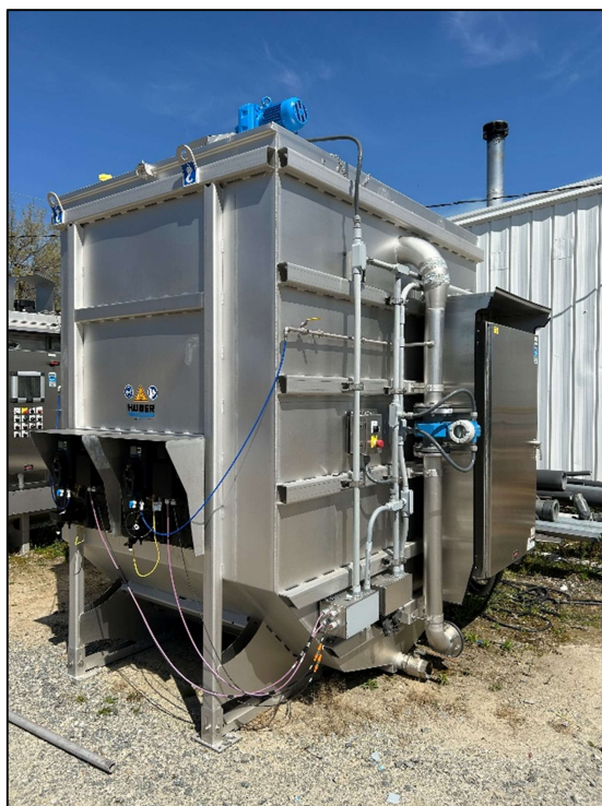
Influent & Turbidity monitoring system Control Panel
