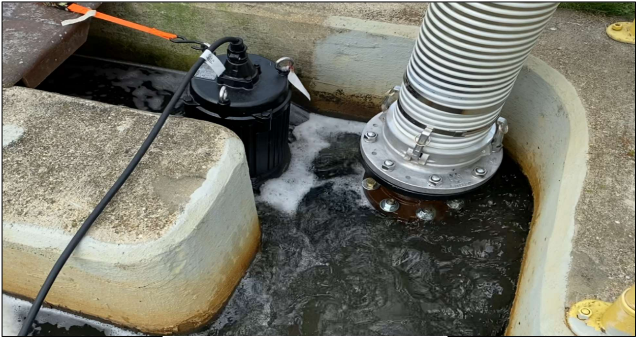
Reference Feed Pump Installation
