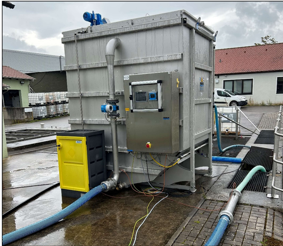
Chemical Dosing Cabinet; Static Mixer
