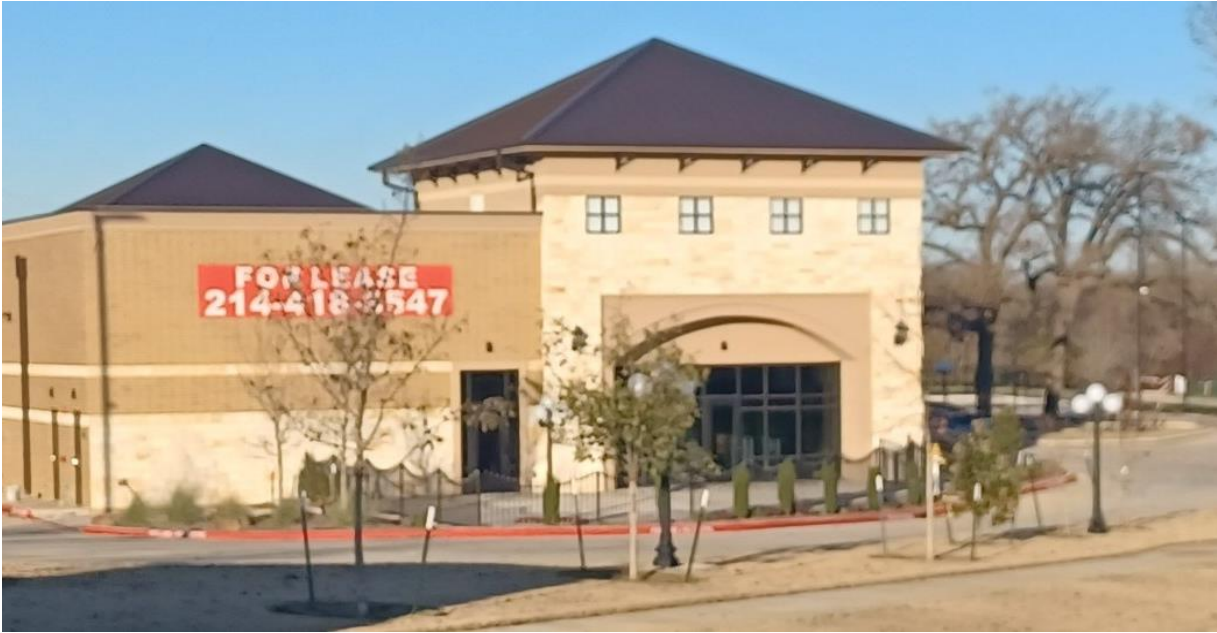
Side of future restaurant tenant at Magnolia Center facing I-35E
