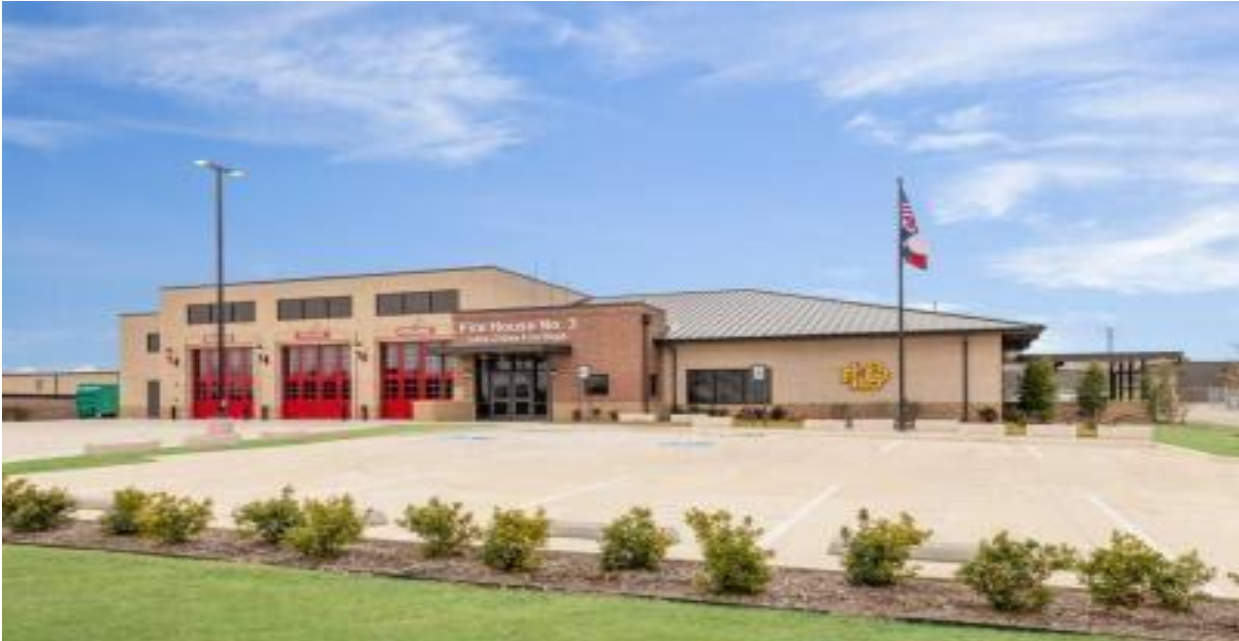
Figure 19: Lake Cities Fire Station #3
