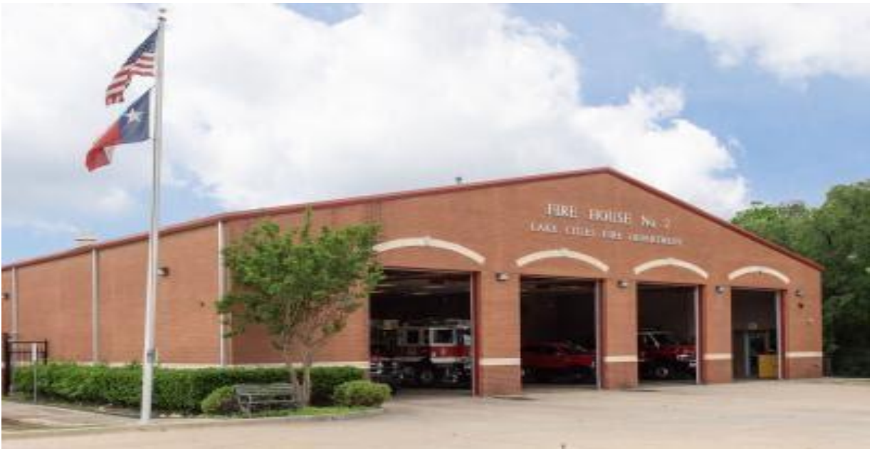
Figure 18: Lake Cities Fire Station #2
