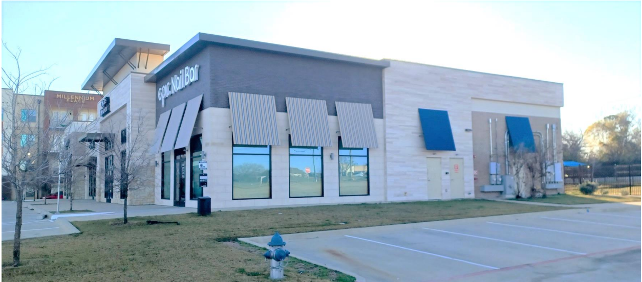
Side of retail tenant at Millennium facing I-35E
