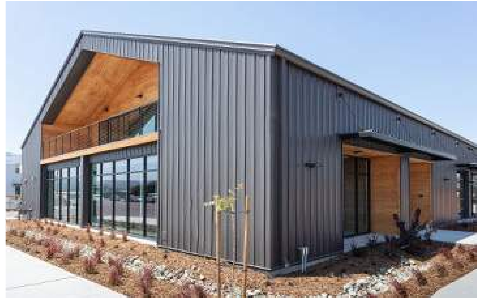
METAL WALL PANELS -WHEELER YARD
