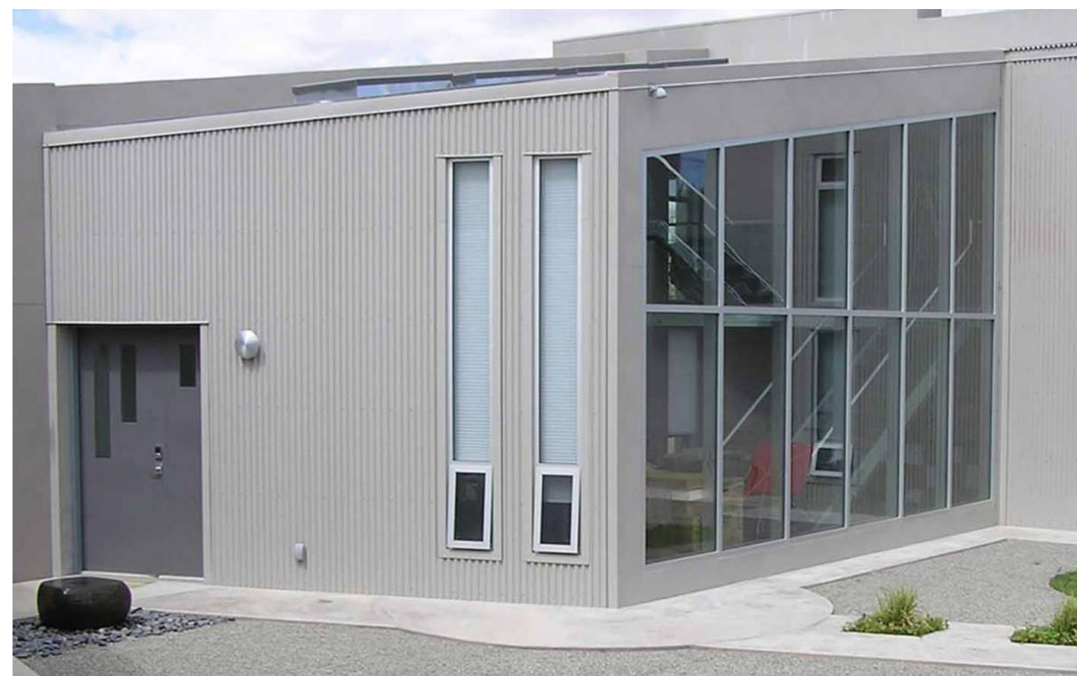
METAL WALL PANELS -WHEELER YARD
