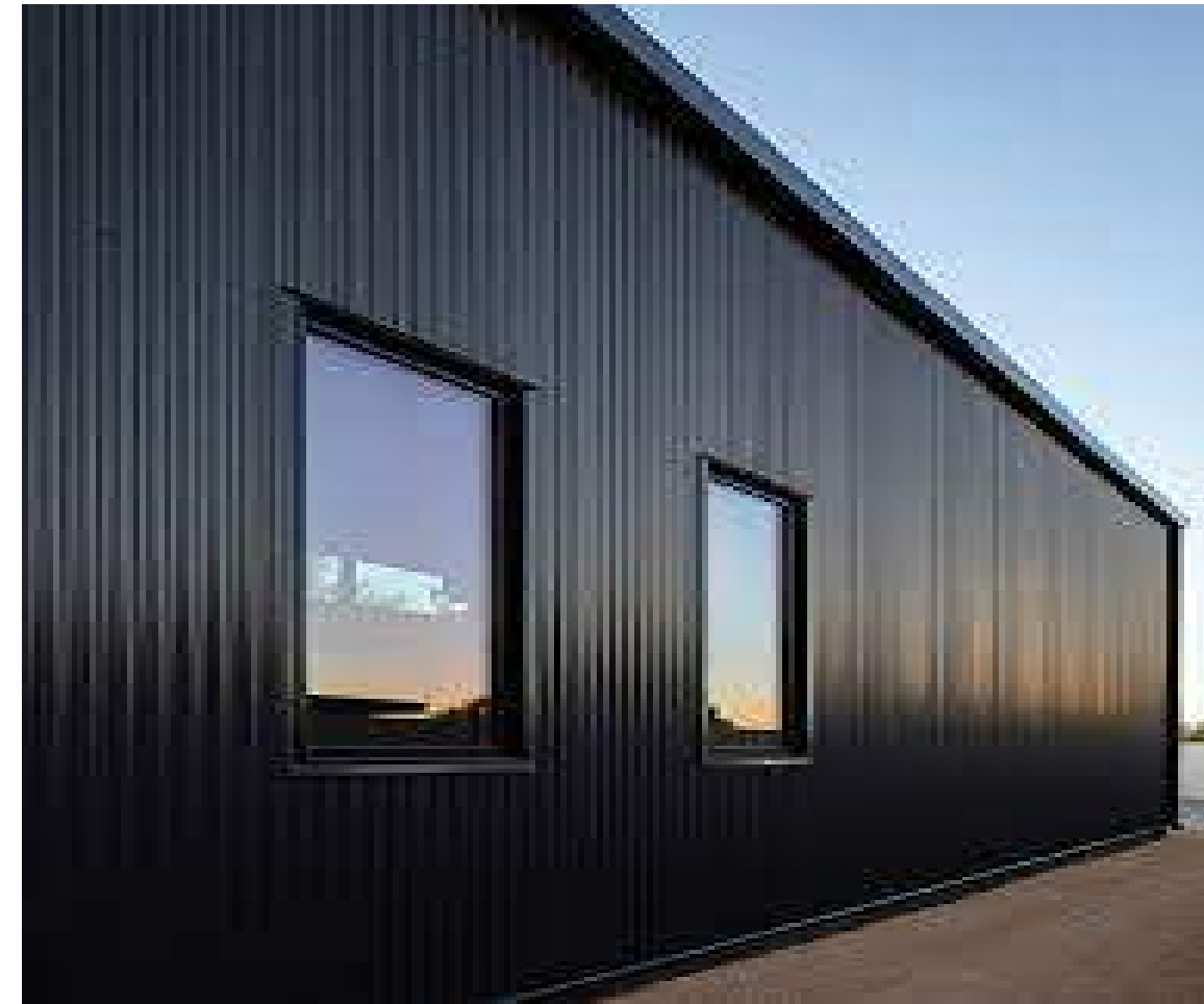
METAL WALL PANELS -WHEELER YARD
