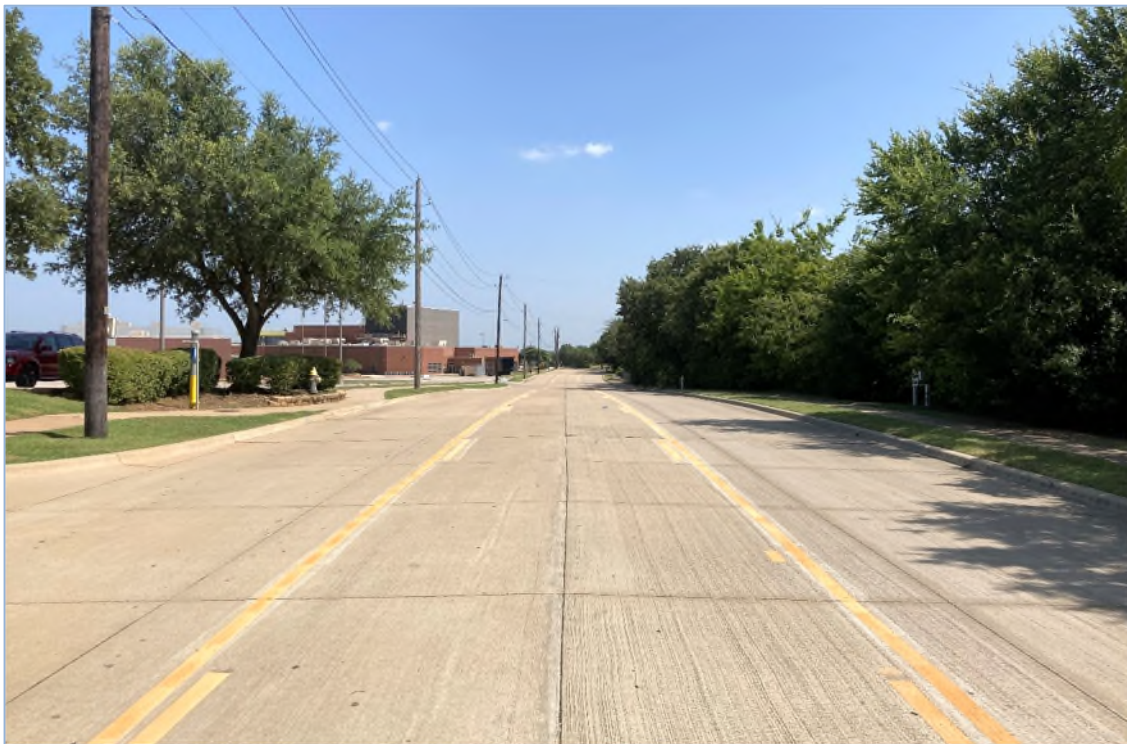
Parkridge Drive - looking south
