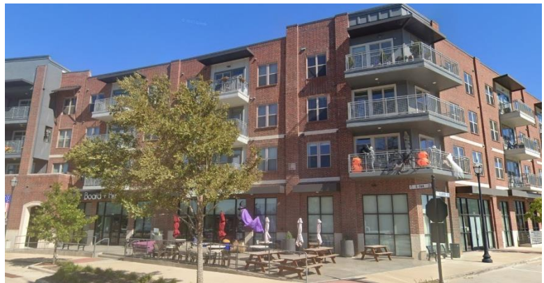
Façade articulation is required through the use of recessed elements, fenestration and expression of structural elements
